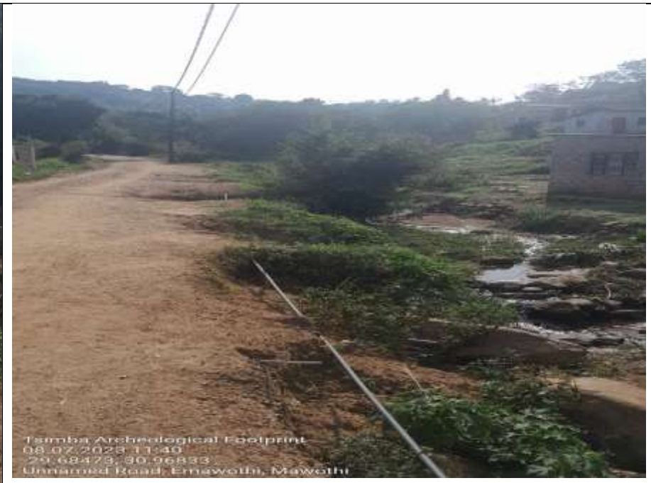
Figure 7: Another portion of the road the sewer collector will be installed
