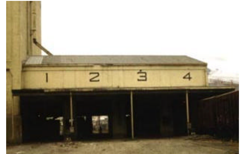
Figure 12: The track shed seen from the north - November 2000 (ref:DW1304)
