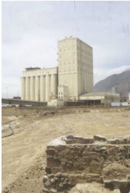
Figure 4: The Grain Elevator seen from the Chavonnes Battery - 1999 (ref: DW0998)
