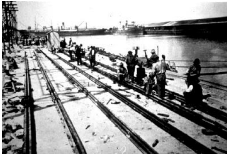
Figure 16: Laying the rails on the collier jetty – 1923 (ref:DW0194)
