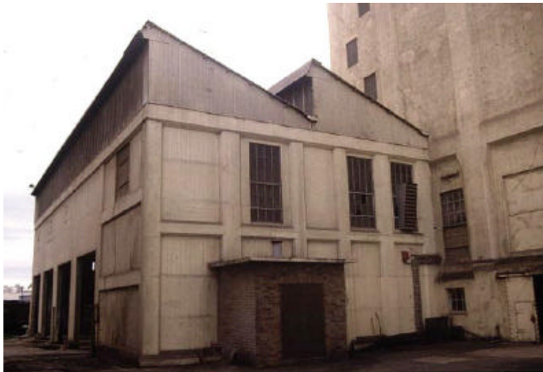
Figure 18: The hydraulic accumulator house – 1995 (ref:DW0056)
