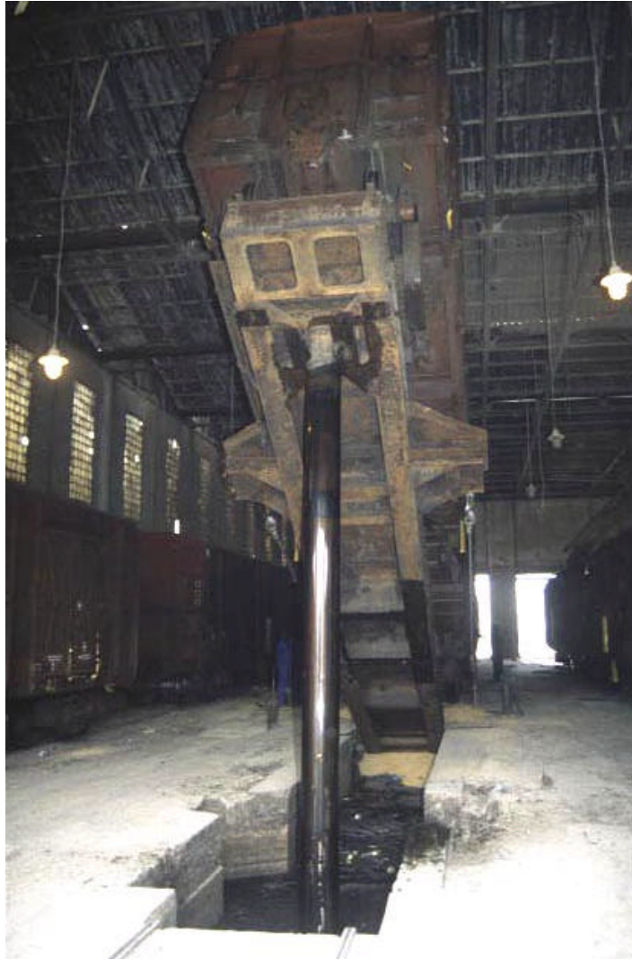
Figure 13: A railway wagon being tipped on track four - November 2000 (ref: DWI325)
