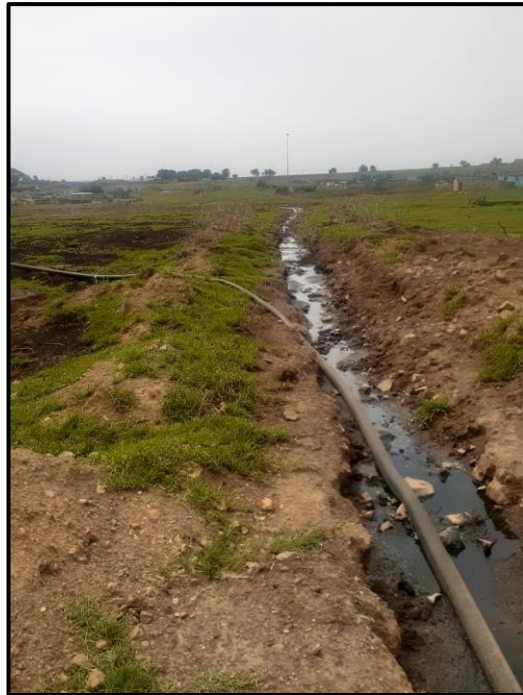
Figure 7. Existing trench for channeling water into the nearby stream.
