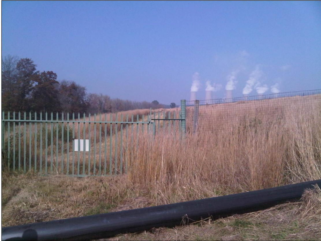
Figure 3 – View of servitude toward Lethabo pump station
