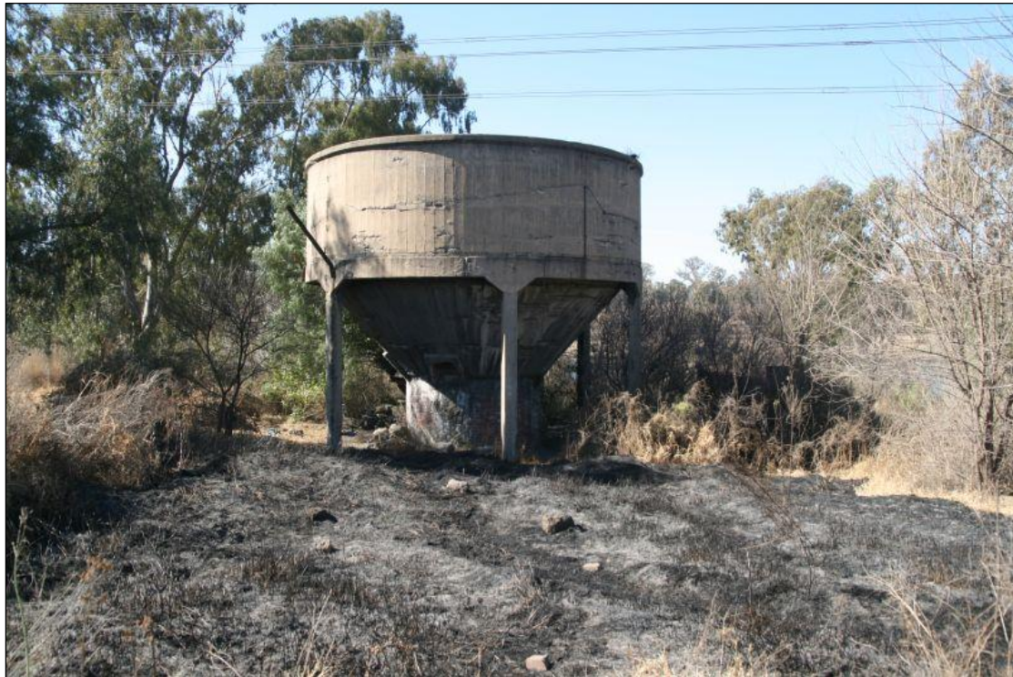
Figure 15 – Brick and concrete structure
