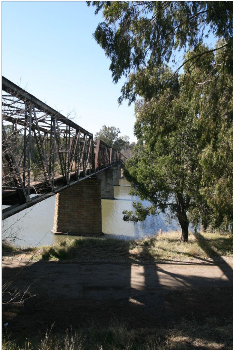
Figure 16 – Brick and concrete structure
