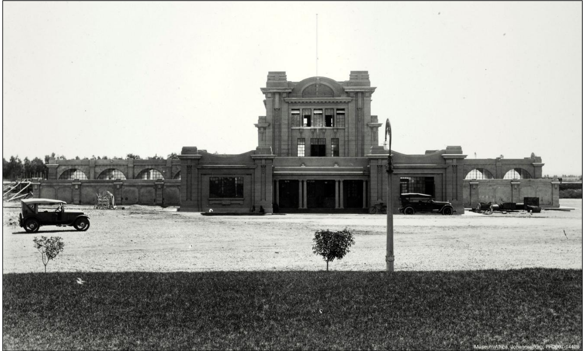
Figure 11 - Historic photograph depicting the construction of the Offices, Laboratory and first Filter Block. The image was taken during 1922 or 1923 (Museum Africa, Images Collection, PH2007-14428).
