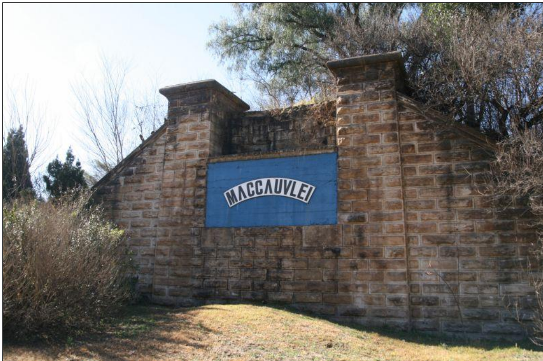
Figure 14 – Stone bridge foundation of RW1
