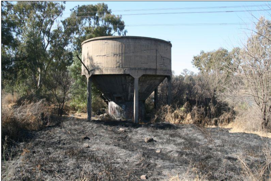
Figure 15 – Brick and concrete structure
