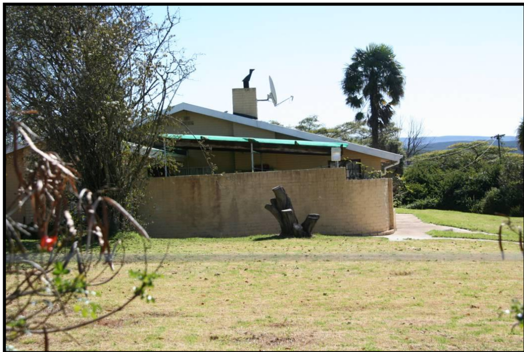
FIG. 10: HOUSE ADJACENT TO THE LANDFILL SITE
