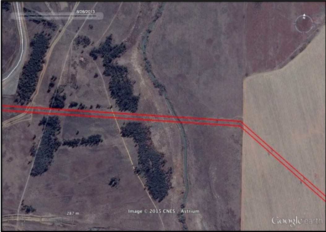
Steenkoolspruit at area where power lines cross over
