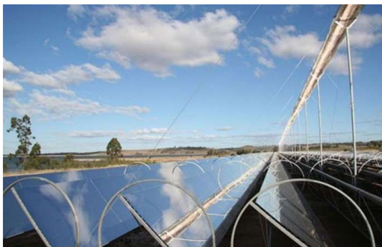
Figure 7: Linear Fresnel Reflector Technology ( social.csptoday.com )
