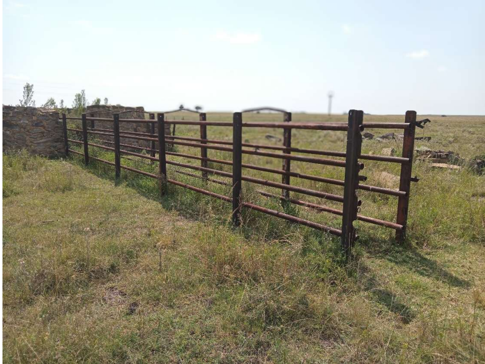
Figure 35: Closer view of the existing cattle race
