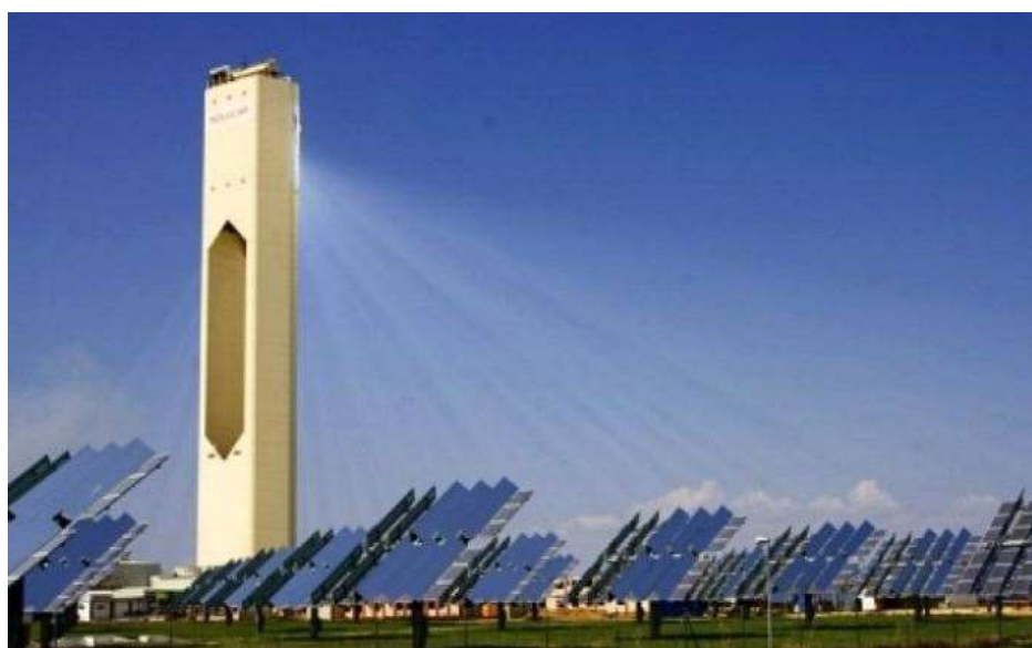
Figure 5: Power Tower Technology (Planta Solar 10, Spain)
