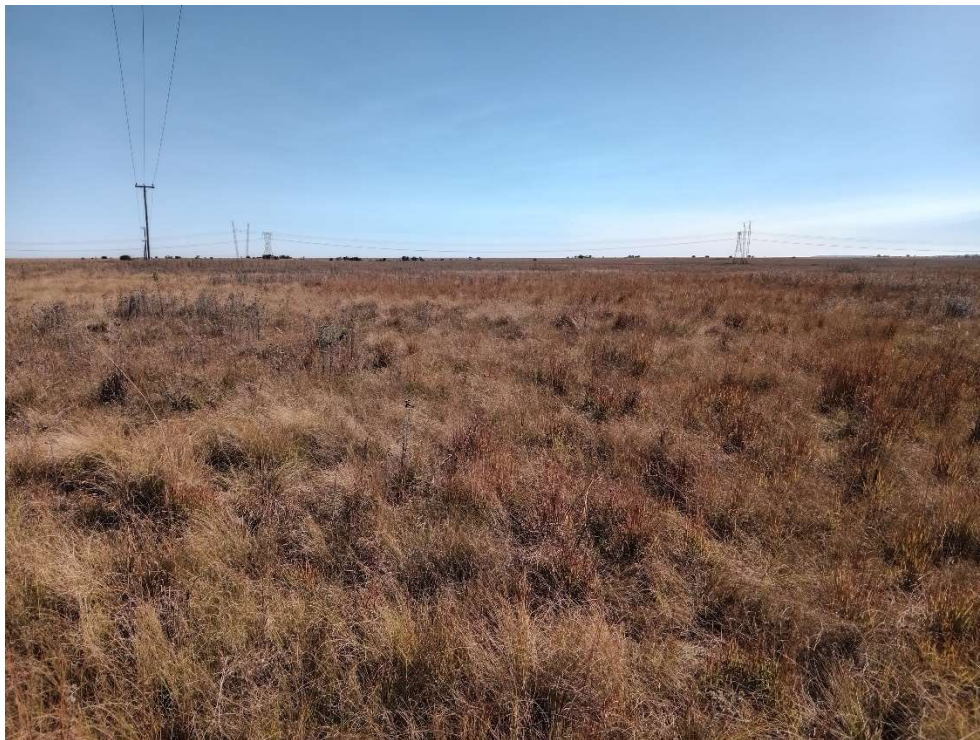
Figure 18: View over the northern section of the longer powerline route option (Alternative 2)
