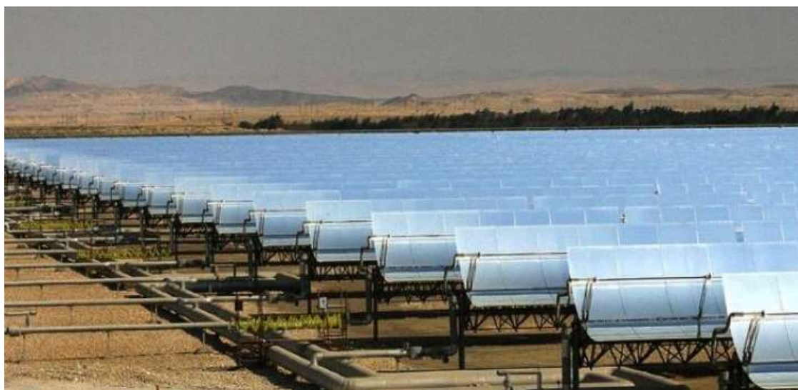
Figure 4: Parabolic Trough Technology ( www.e-education.psu.edu )
