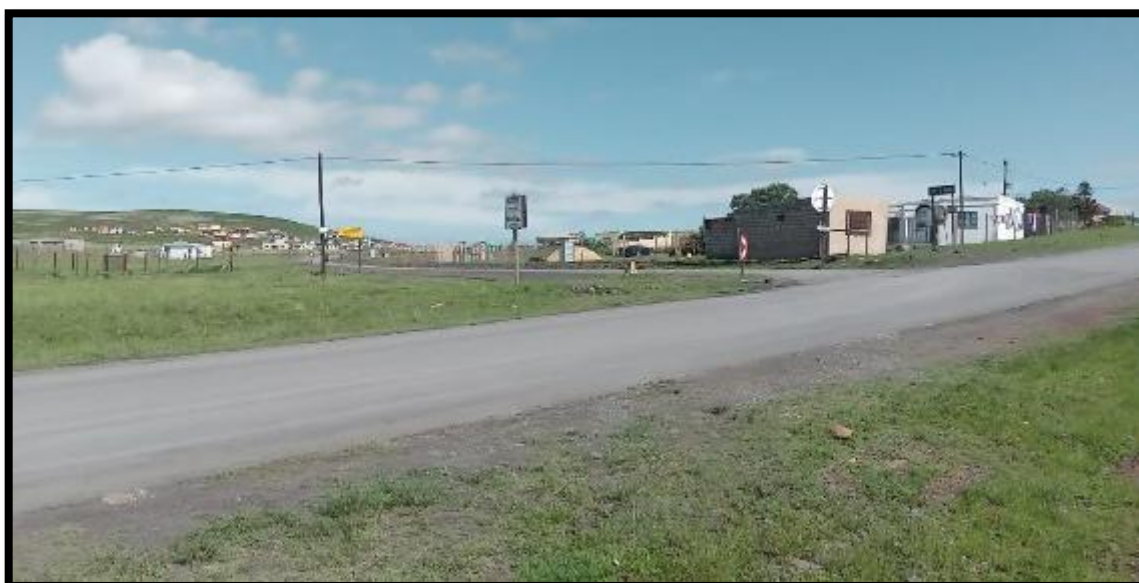
Figure 9. Entrance to Gugwini Village. All the buildings adjacent to the road are younger than 60 years old.
