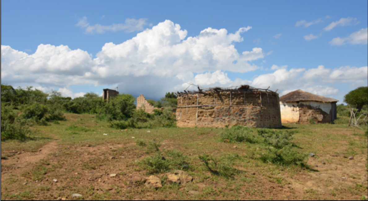
Figure 18. Guswini road upgrade
