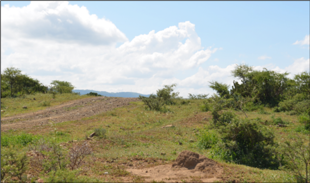
Figure 17. Guswini road upgrade
