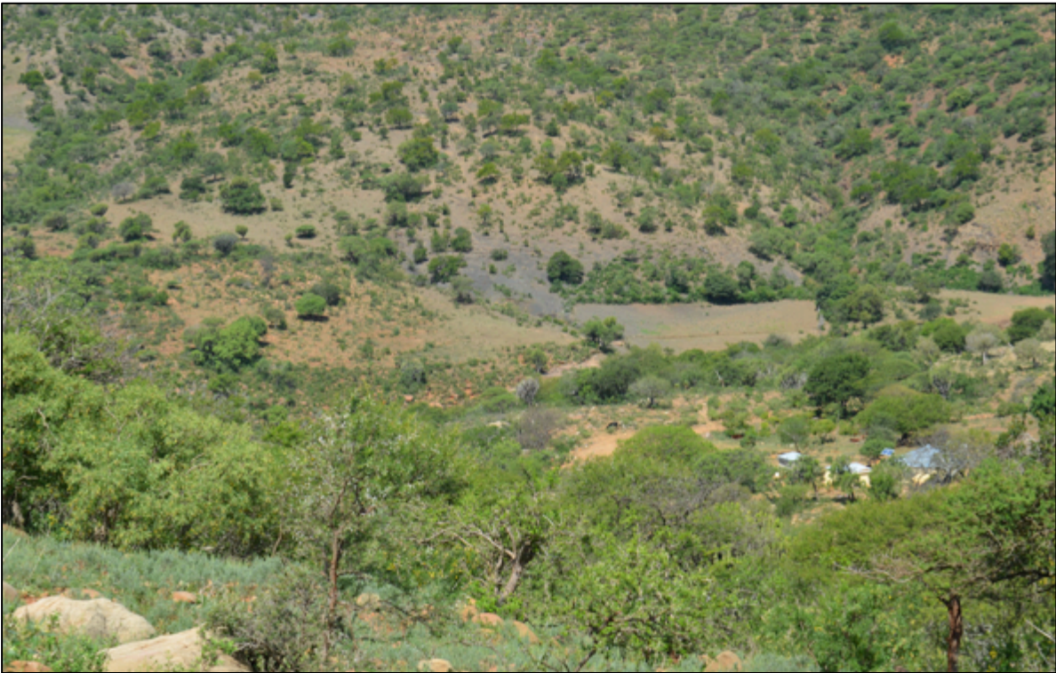
Figure 16. Guswini road upgrade
