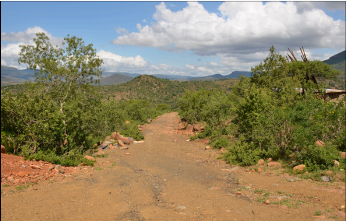
Figure 14. Guswini road upgrade
