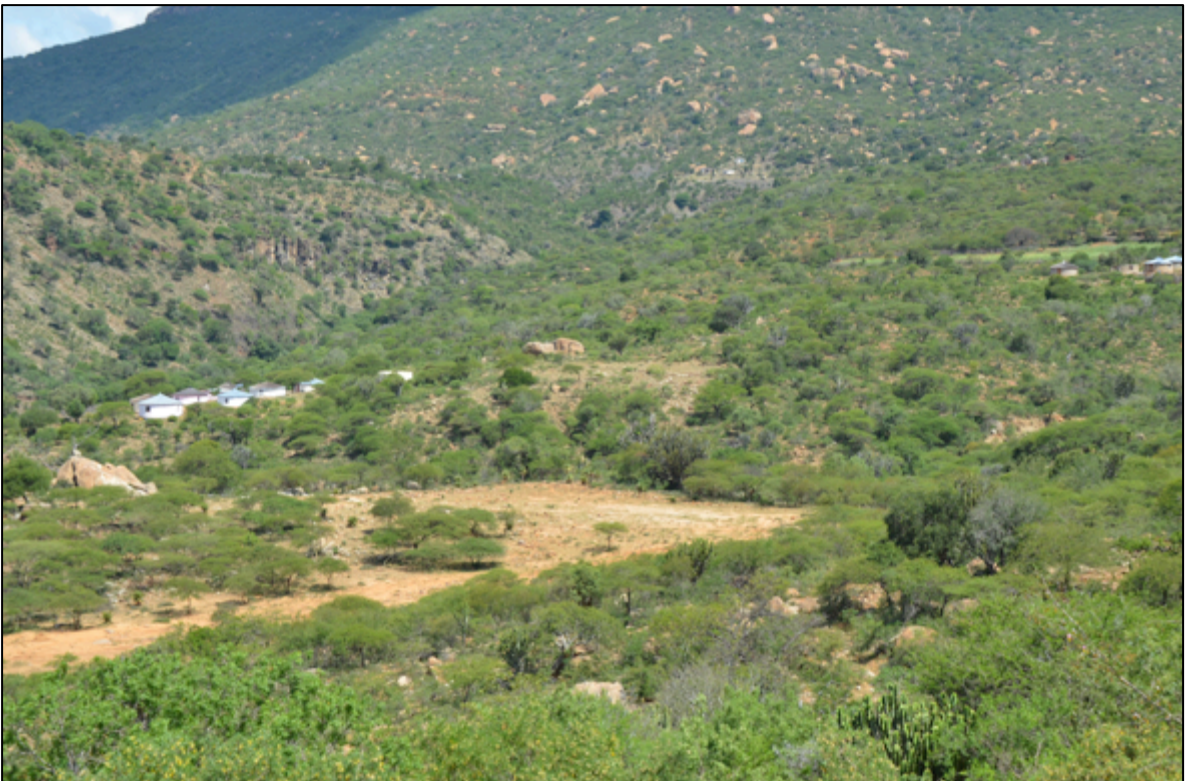
Figure 15. Guswini road upgrade
