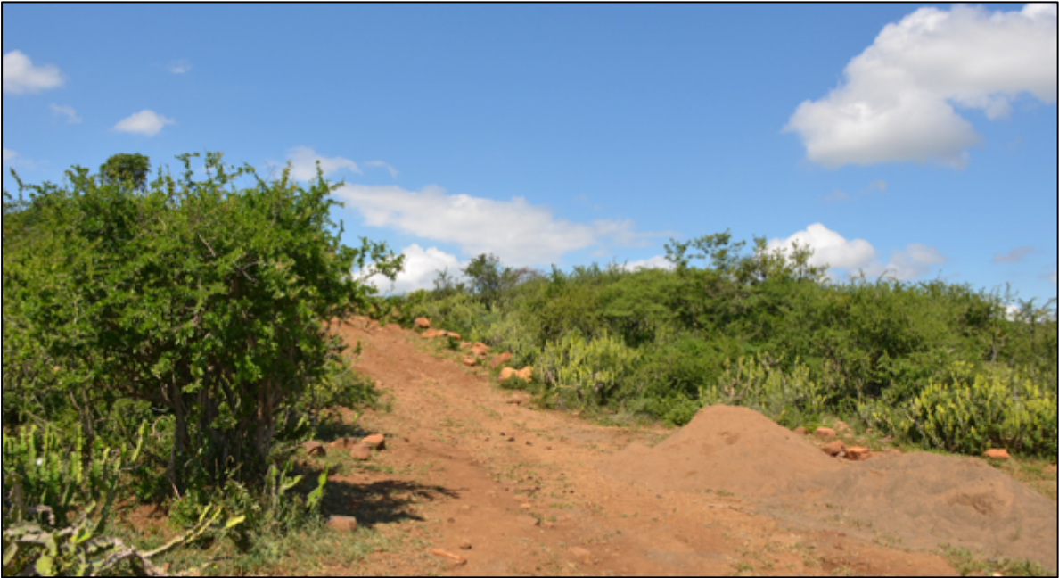
Figure 19. Guswini road upgrade
