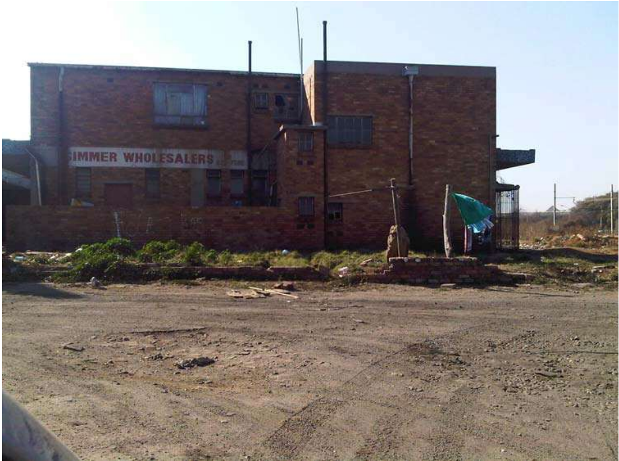
Figure 10: West elevation (taken in 2010 by SEF).
