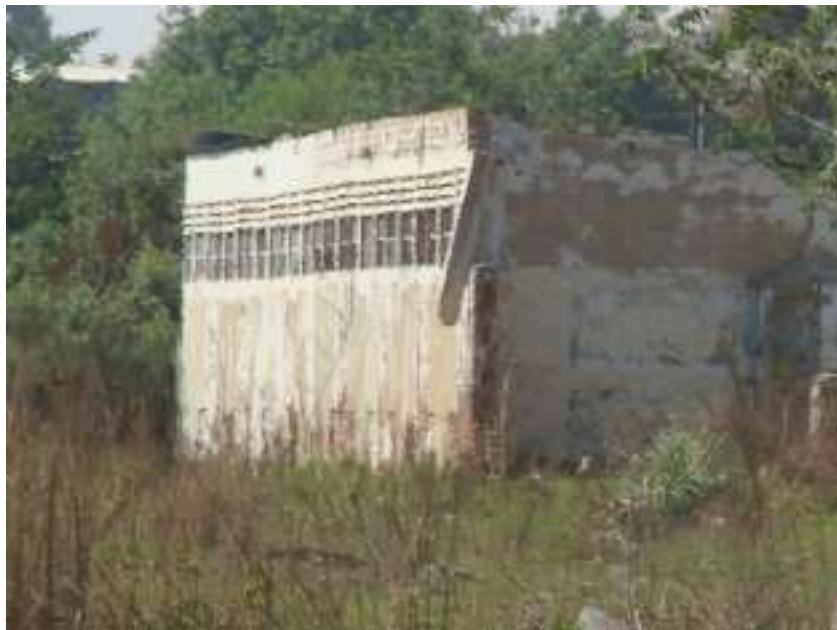
Figure 15: More demolished structures in the area.
