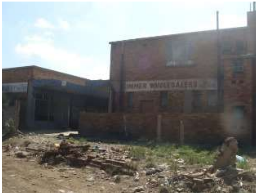
Figure 11: Photo taken in 2013. Note the vandalism evident with windows broken etc.
