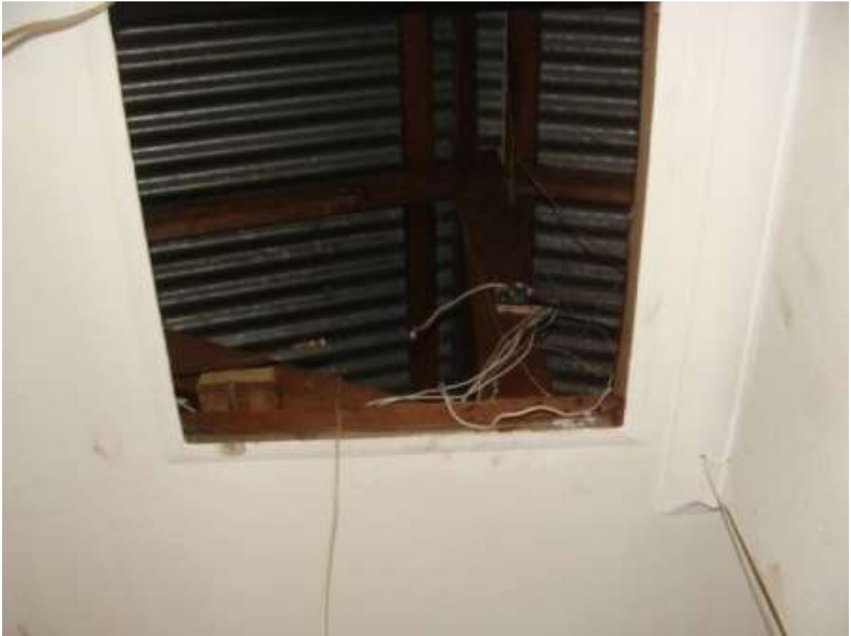
Figure 14: View of a section of the roofing. This is modern.
