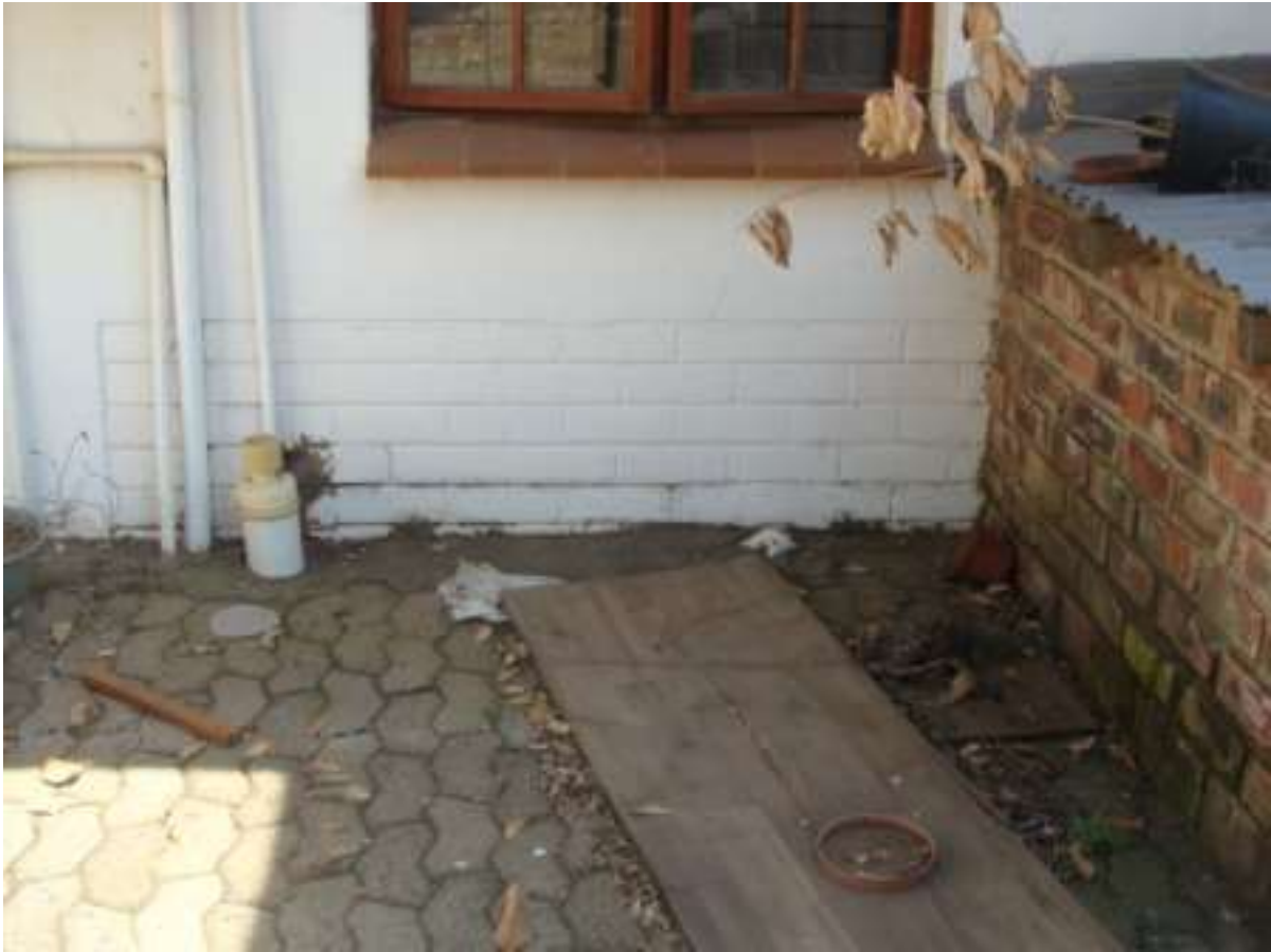
Figure 12: A section of plastered over bricks that could be the remnants of an earlier structure.
