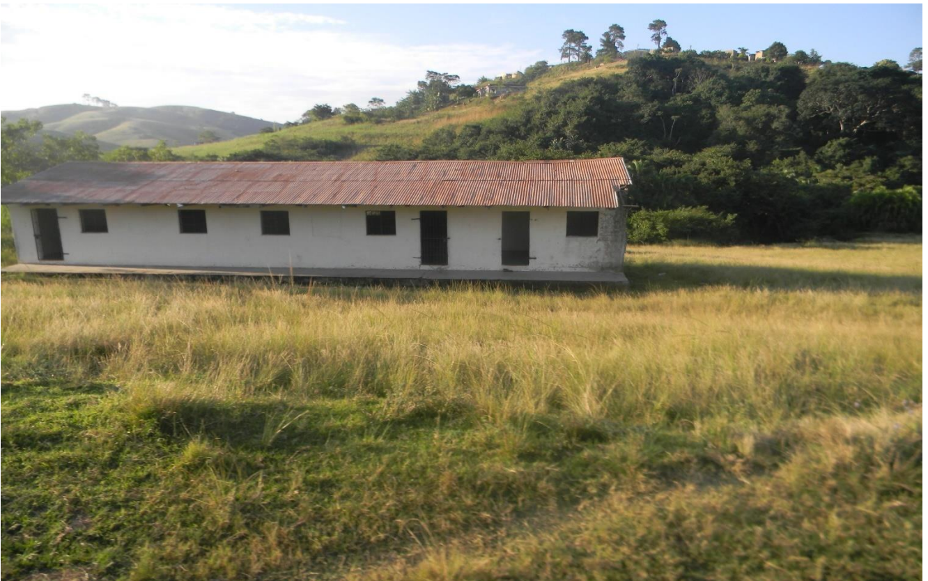
Plate 21: showing a building which is older than 60 years
