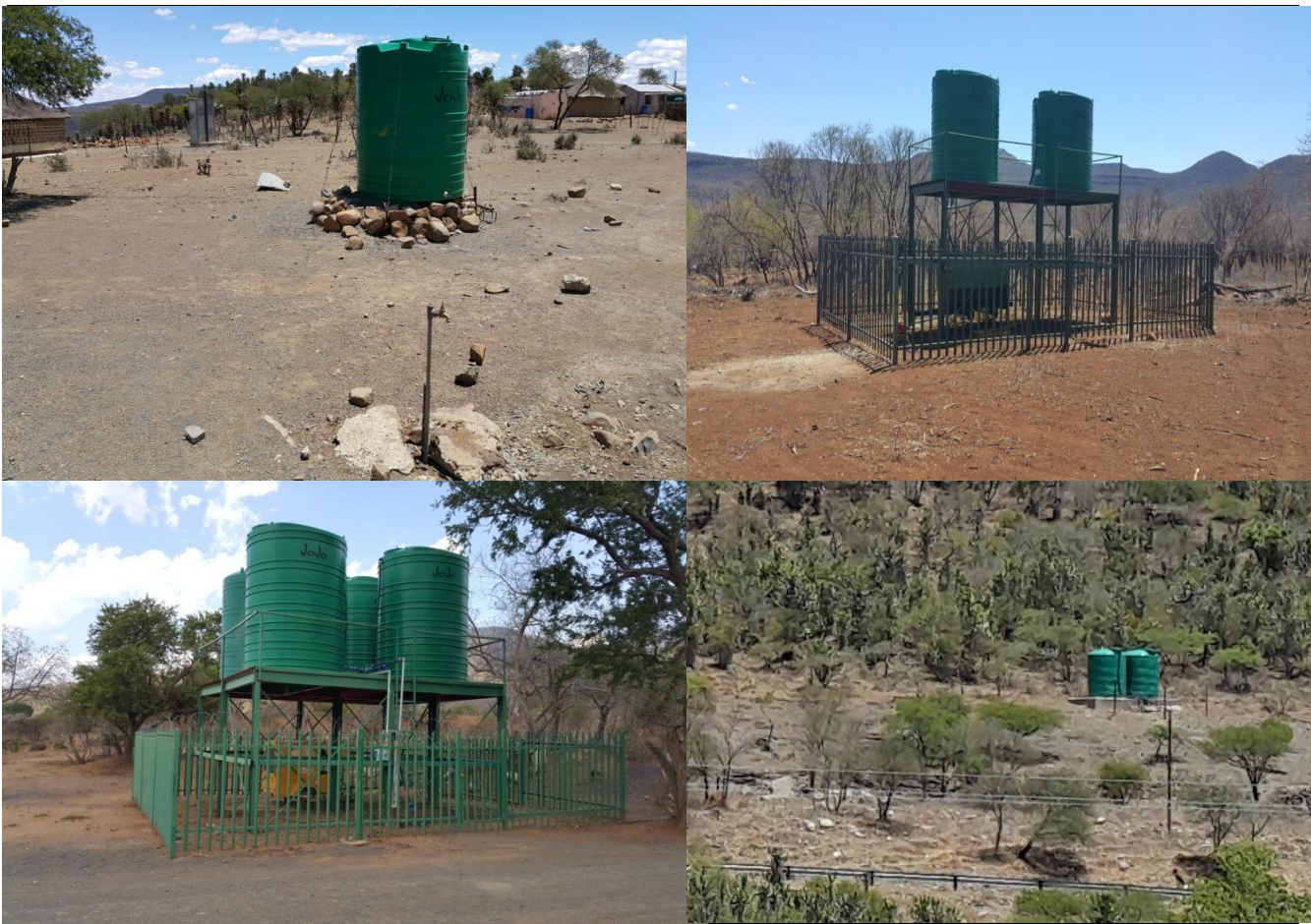
Figure 8- The existing JoJo water storage tanks
