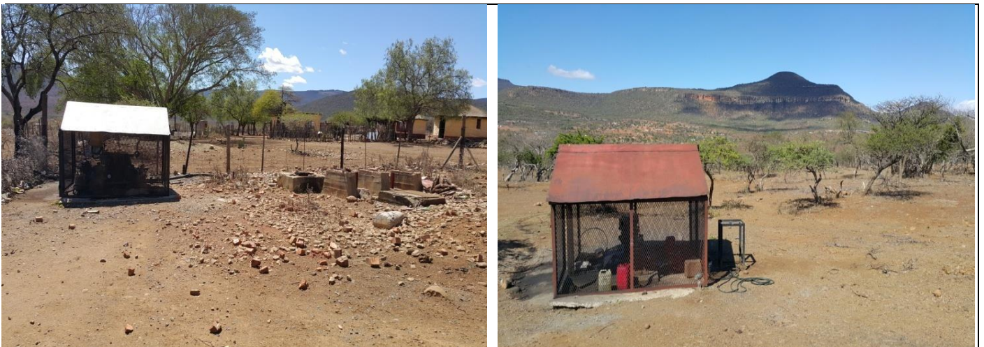
Figure 10- Diesel engines that assist with pumping of water from reservoirs and boreholes to communities
