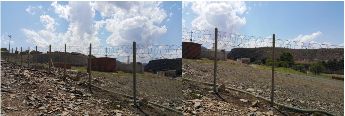
Figure 7-Existing Keates Drift Water Works reservoirs
