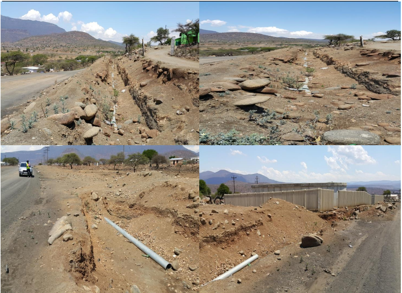
Figure 9-Water trenches along the D1268 Road
