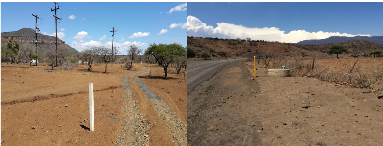
Figure 3- Existing water pipeline markers (yellow and white cement marker)
