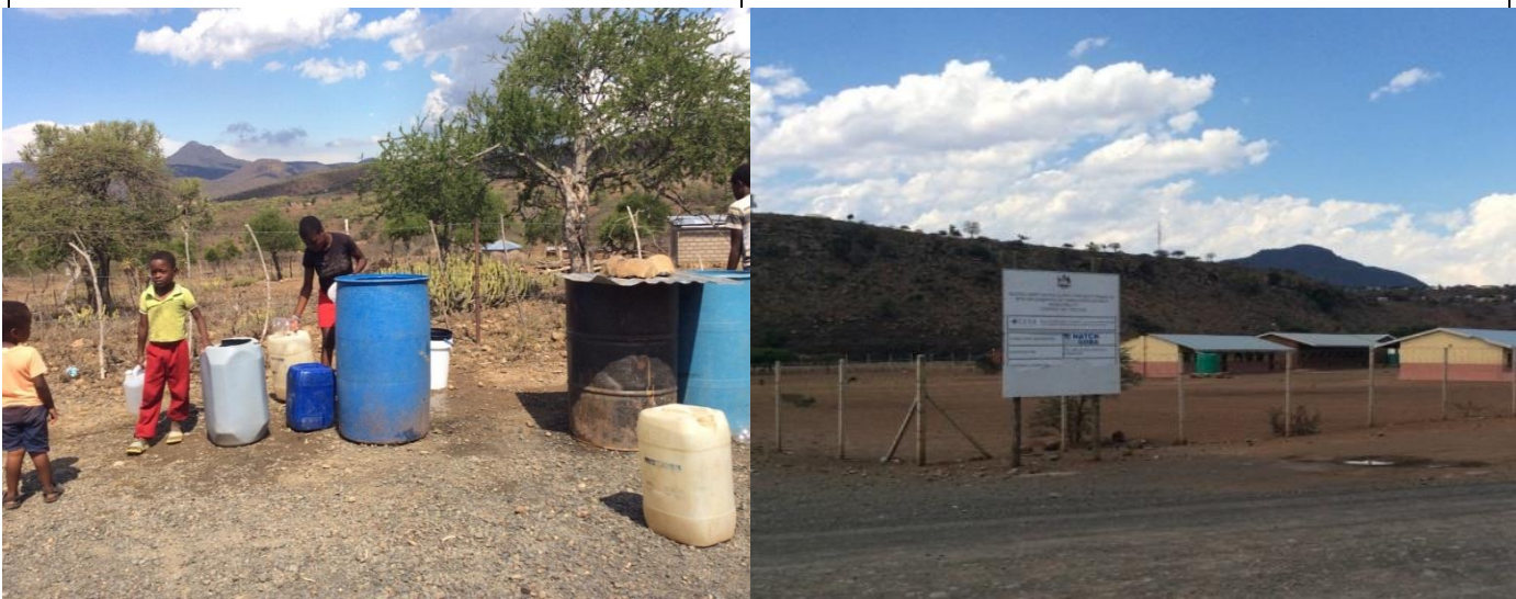
Figure 5- Above are existing water distribution pipelines within villages. Below (left) is current water collection point to affected communities. Below and right is the project communication board.
