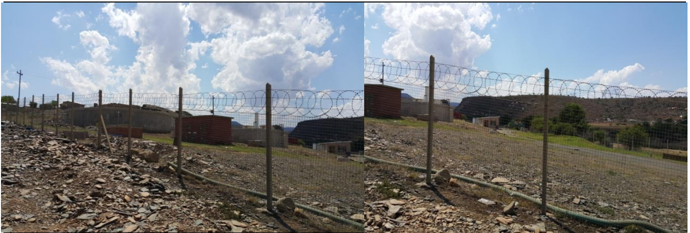
Figure 7-Existing Keates Drift Water Works reservoirs
