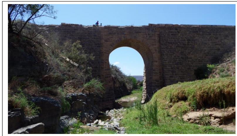
Figure 8: The bridge from the west. (Photo: The Author)
