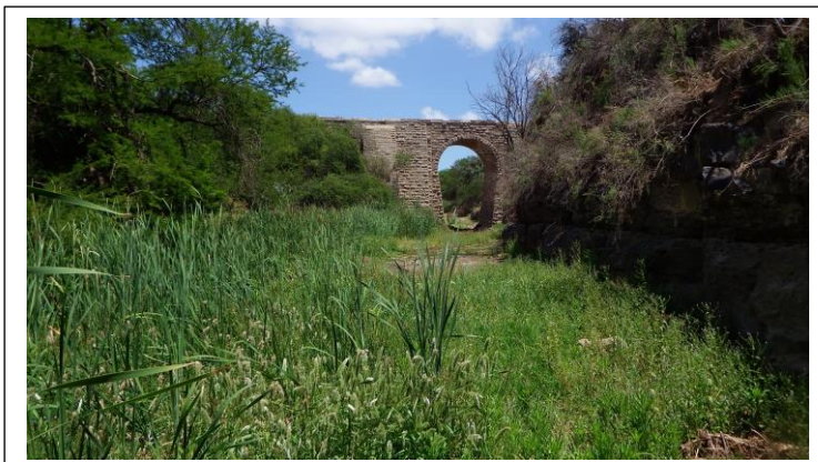
Figure 27: Bridge DR02481 (Photo: The Author)
