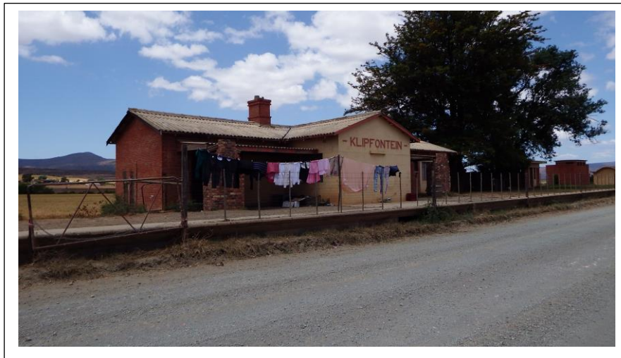
Figure 2: The old Klipfontein Railway Station on the DR02481, now used as a house. (Photo: The Author)
