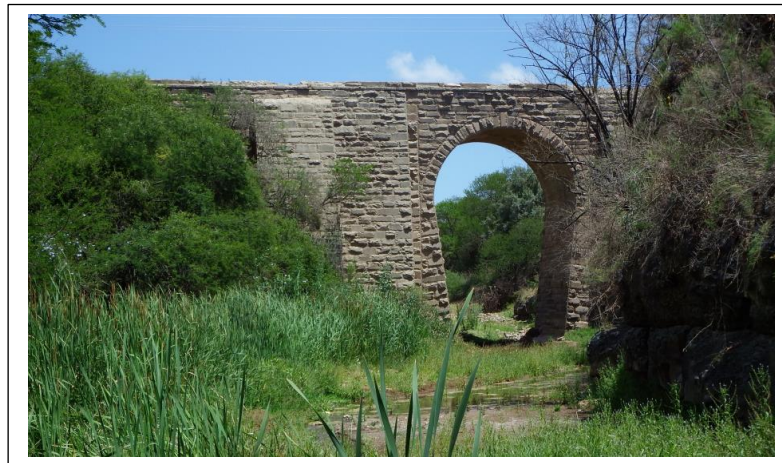
Figure 14: Bridge from the east. (Photo: The Author)
