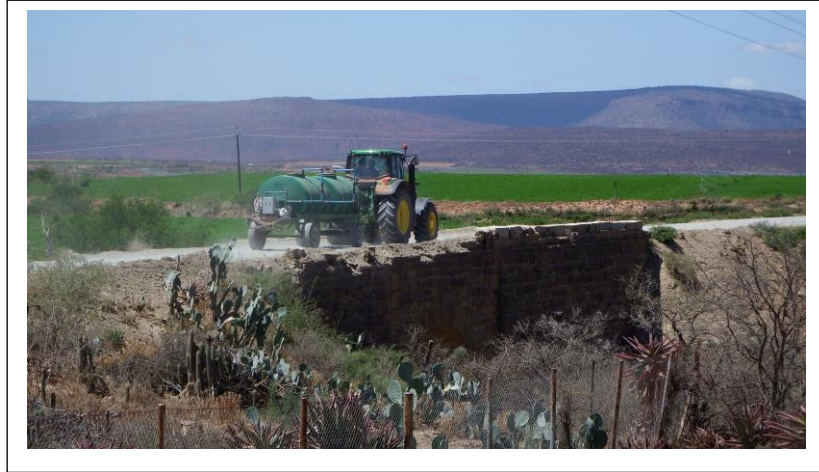
Figure 4: Tractor crossing the bridge. (Photo: The Author)
