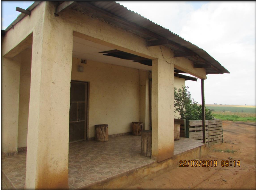
Figure 11: One of the other farm structures on the property.
