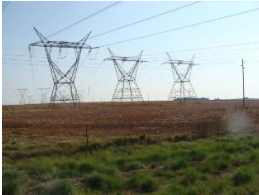
Figure 3: Existing powerlines in area crossing over ploughed fields.
