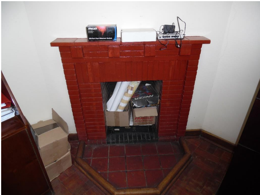
Photograph 10: Victoria West Magistrates Court: Fireplace Detail
