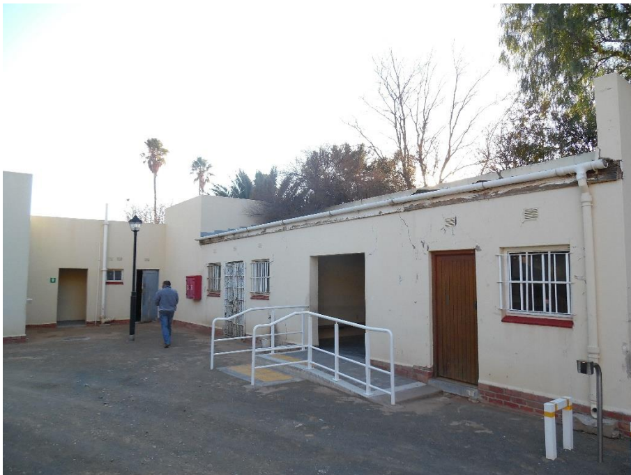
Photograph 20: Outbuilding (to be demolished and reconstructed, exact footprint)
