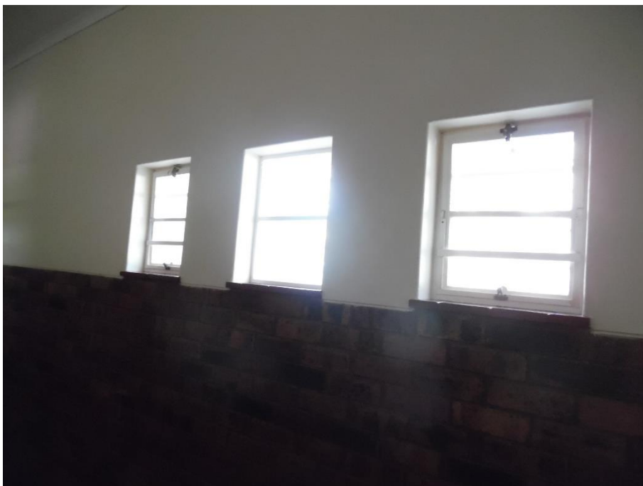
Photograph 12: Victoria West: Steel Window Detail
