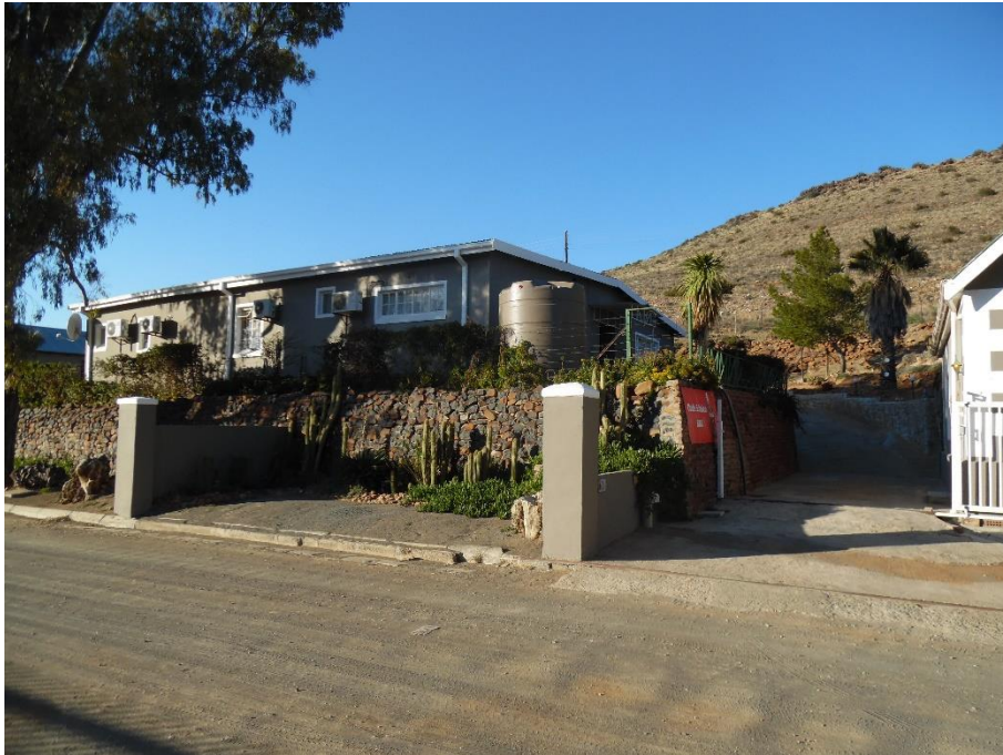
Photograph 23: Victoria West Magistrates Court: Structure Opposite (South)
