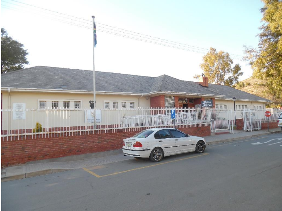
Photograph 1: Victoria West Magistrates Court: West Elevation
