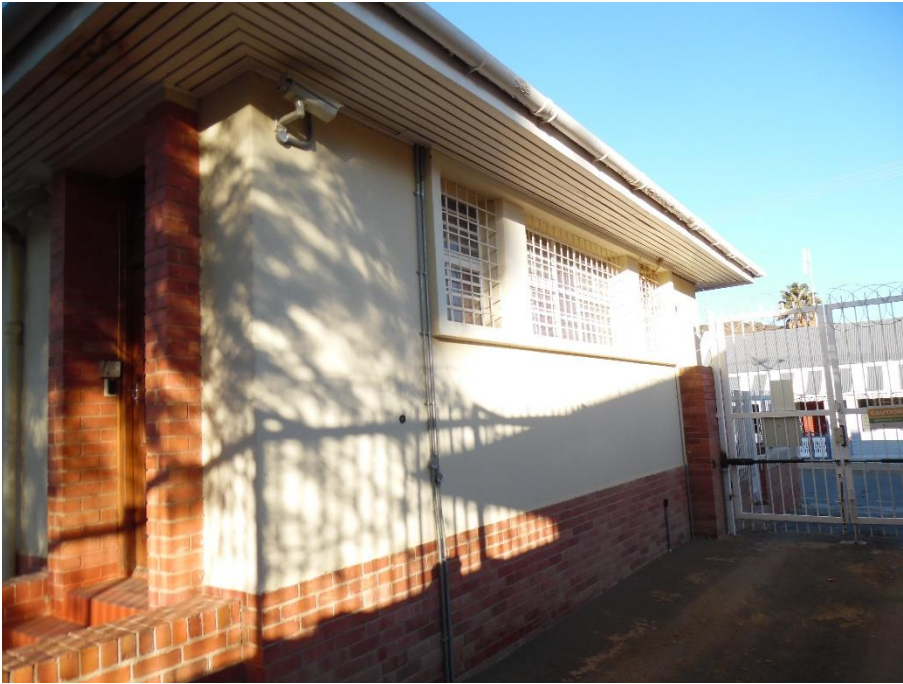
Photograph 3: Victoria West Magistrates Court: North Elevation
