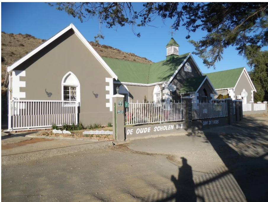
Photograph 22: Victoria West Magistrates Court: Structure Opposite (South)
