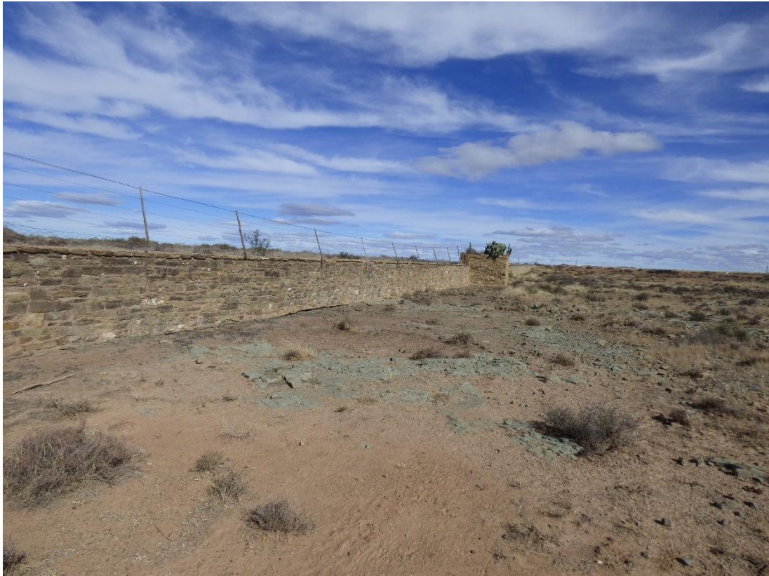
Figure 36: Part of the Site 016 retaining wall (courtesy Ubique Heritage Consultants).
