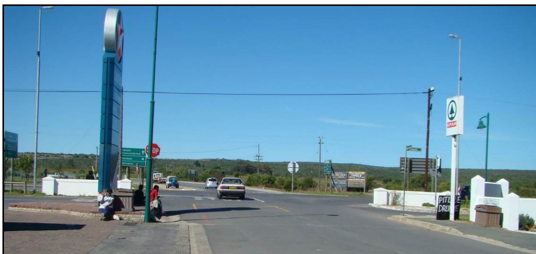
Plate 3: View of the intersection at Stanford which would be replaced with a traffic circle.
