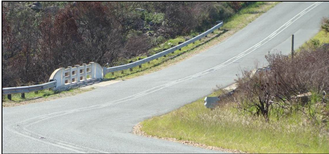
Plate 2: View of the Vogelgat Bridge which would be replaced by realigning the road to the south of the existing alignment (preferred alternative).
