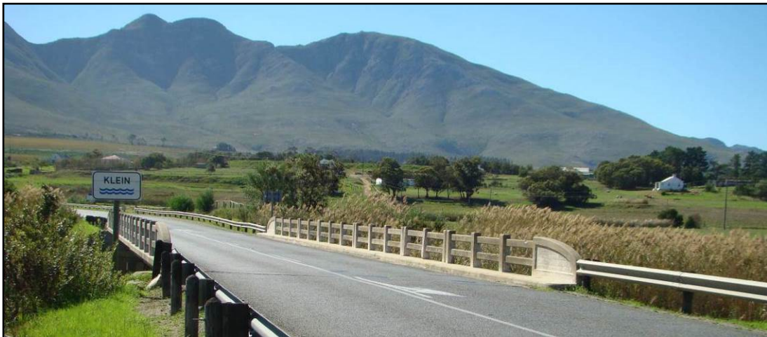
Plate 3: View of the Klein River Bridge which would be replaced with a new bridge on a new alignment to the west of the existing bridge (preferred alternative).
