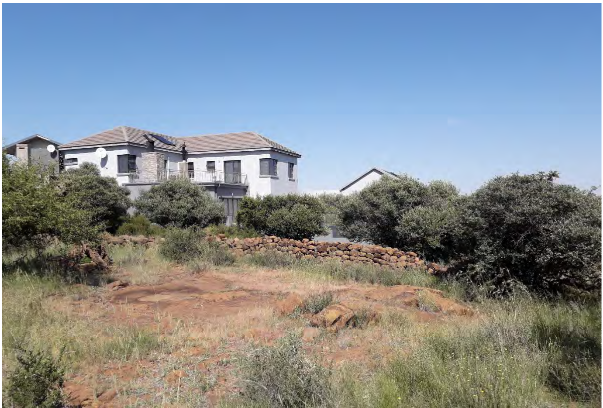
Figure 4: Section of wall leading immediately up to the subject property (right)
