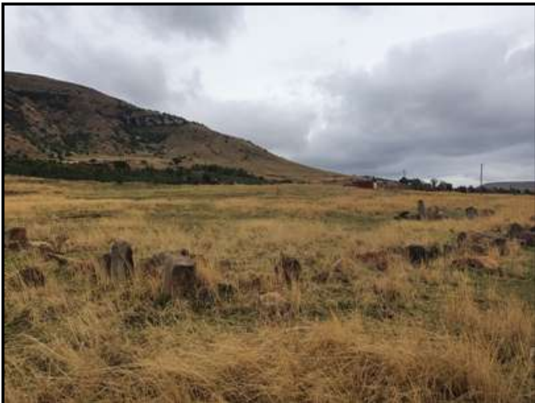
FIG. 8: FOUNDATIONS OF STONE WALLING
