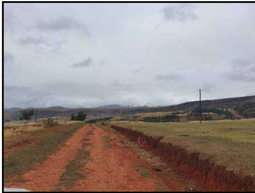
FIG. 4: VIEWS ALONG THE PROPOSED ROAD UPGRADE
