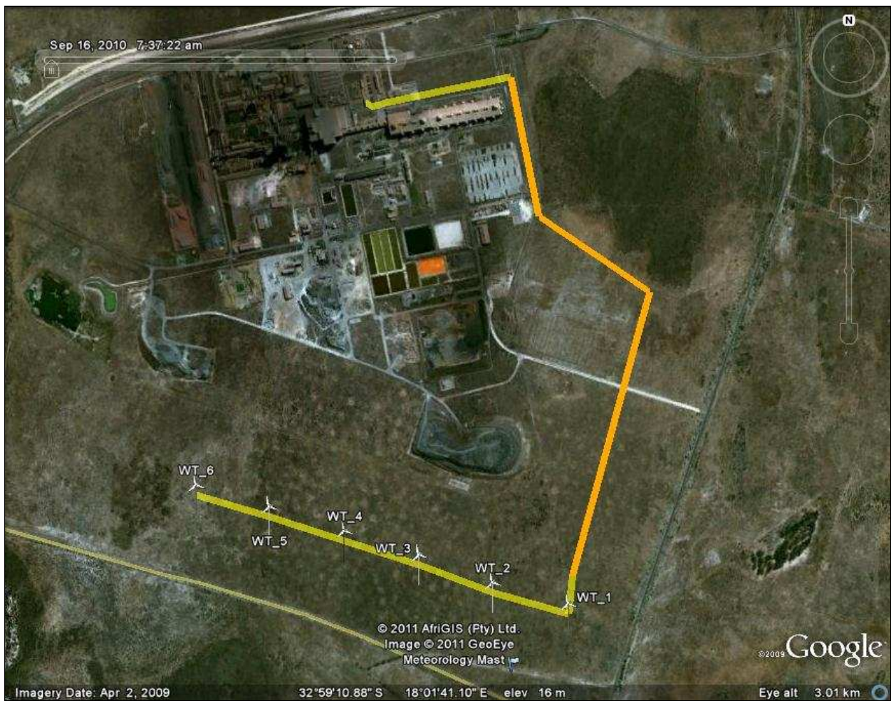
Figure 2: Aerial photograph showing the layout of the proposed WEF. The yellow lines denote subsurface power lines and the orange an above ground power line. The six turbine positions are also shown.
