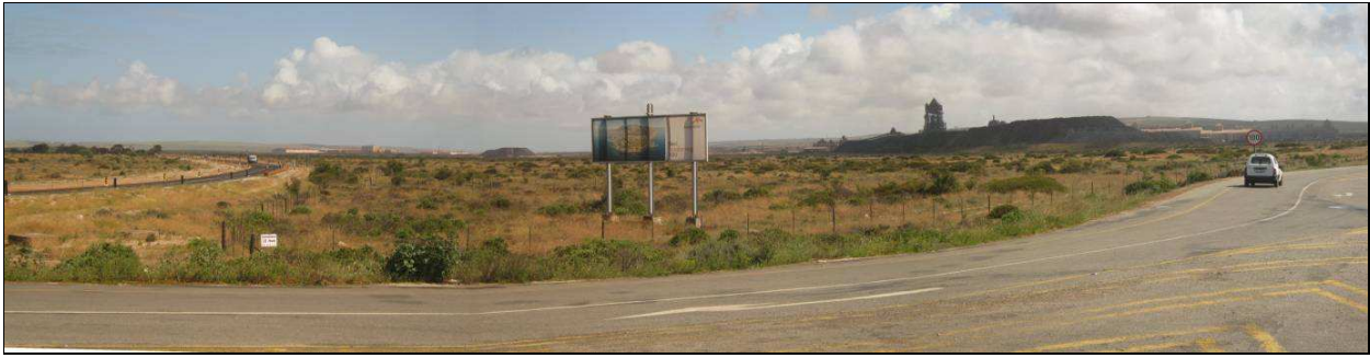
Figure 15: View towards the northwest and north showing the two roads that pass alongside the site. The turbines would be situated approximately behind the advertisement board. Saldanha Steel is visible on the right and other large warehouses in the Port area are visible in the background to the left.
