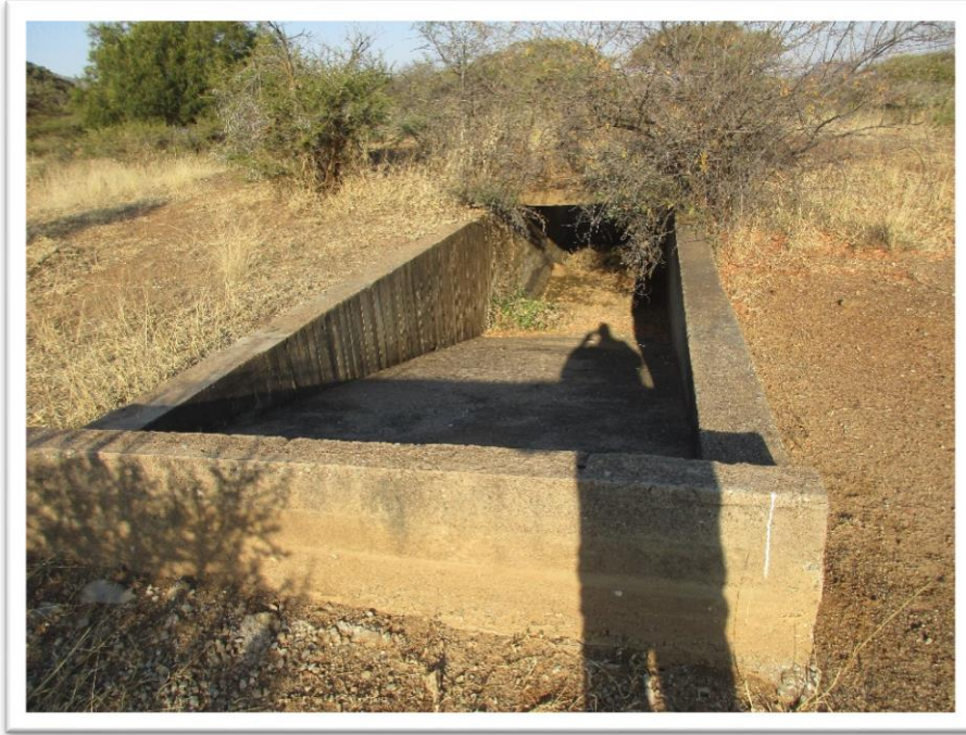
Figure 20: Concrete structure, part of a processing plant (Site PM5).
