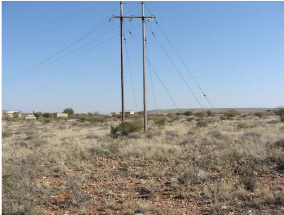
Figure 16 General view of area where both routes end at the proposed Groblershoop Substation.
