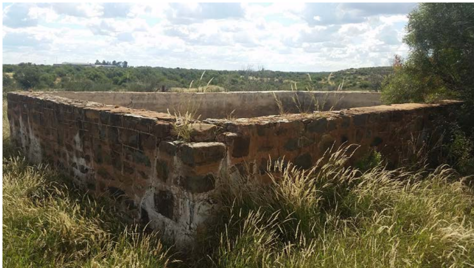
Figure 45: Water reservoir (dressed stone and cement) near the dairy
