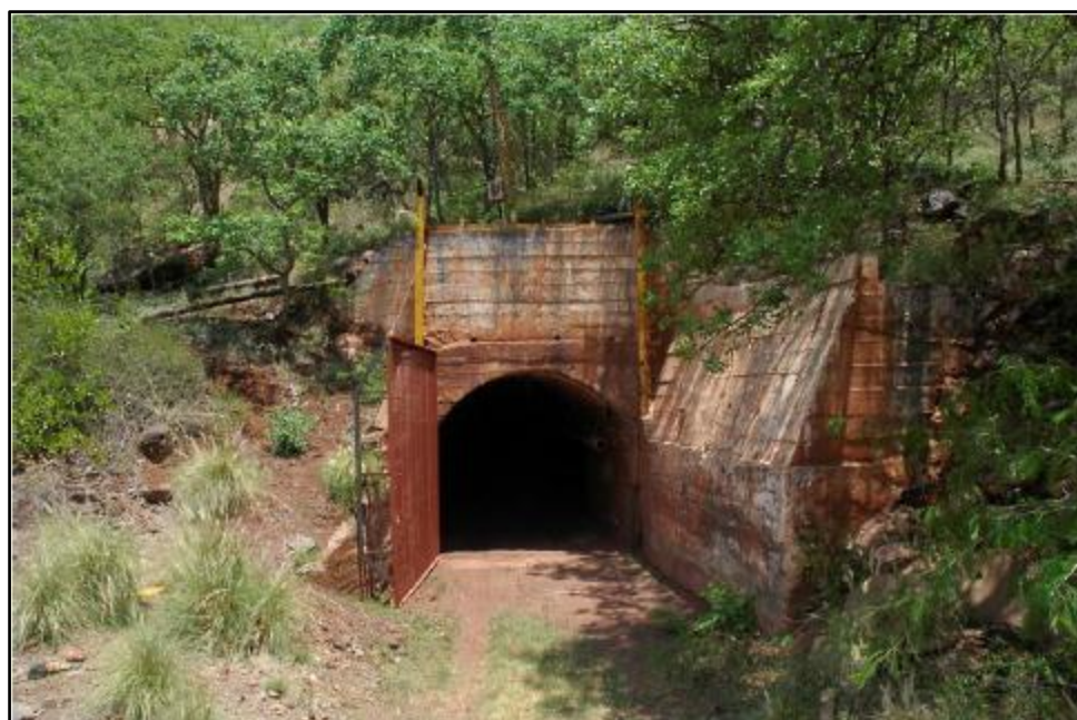
Figure 5 – Entrance to the Mostert Tunnel (Cairncross, 2011)
