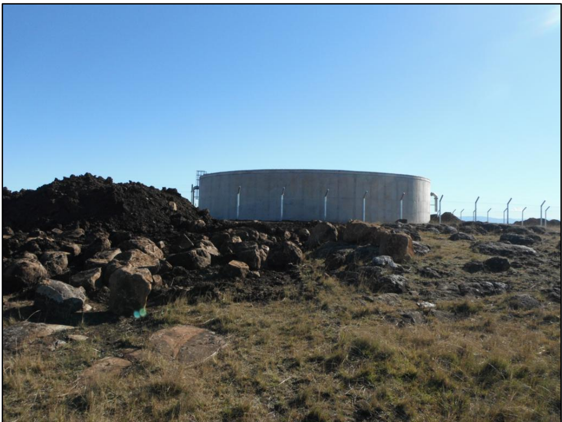
Figure 5 – Construction activity at reservoir R11 as part of construction in Phase 1
