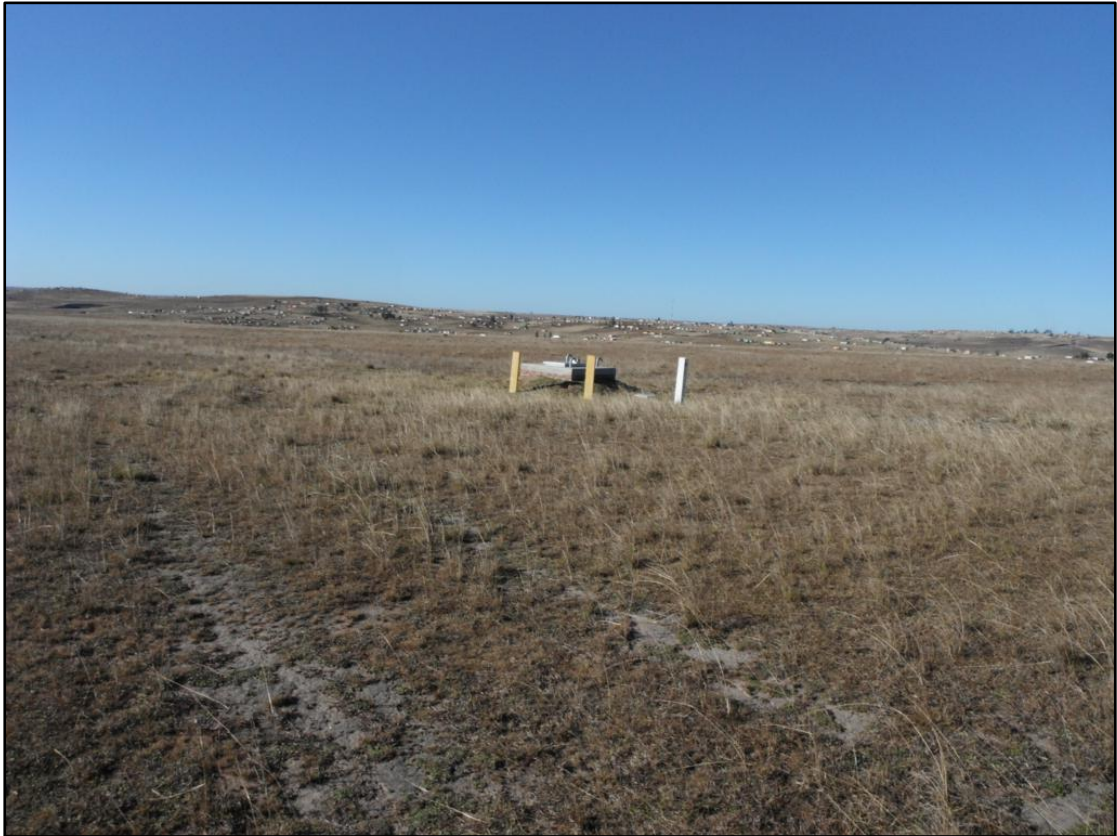
Figure 4 – Reservoir R1 – Already installed during first Phase of the project
