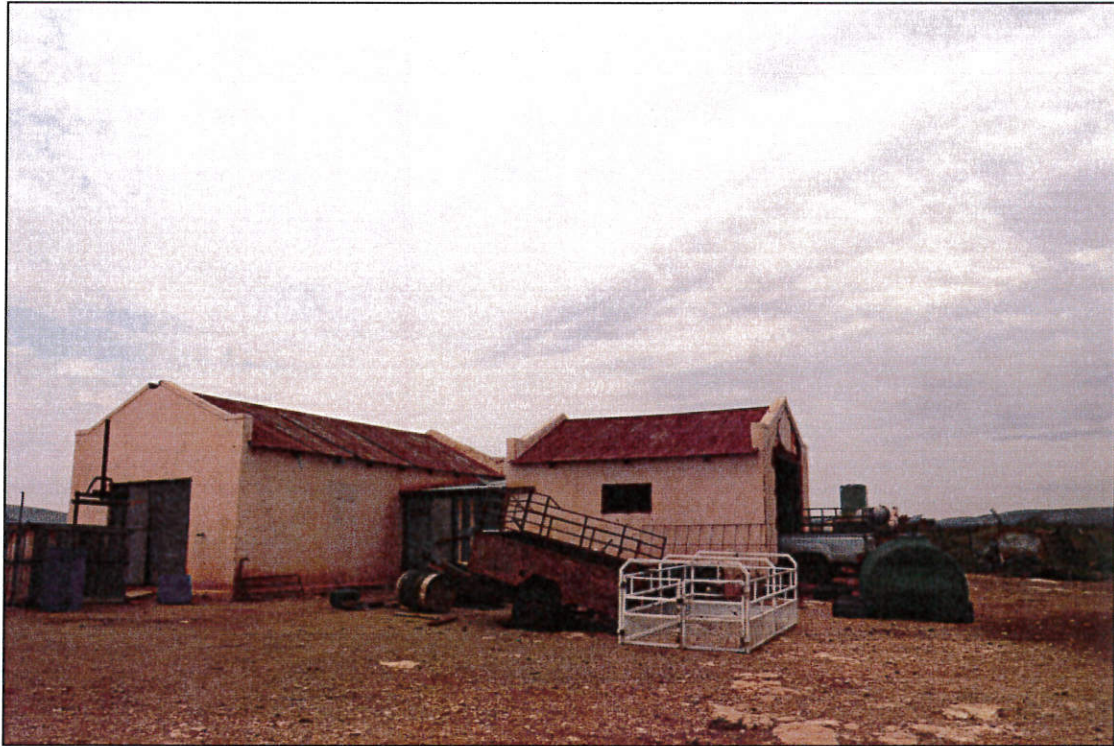
Figure 51. Old homestead outbuildings
