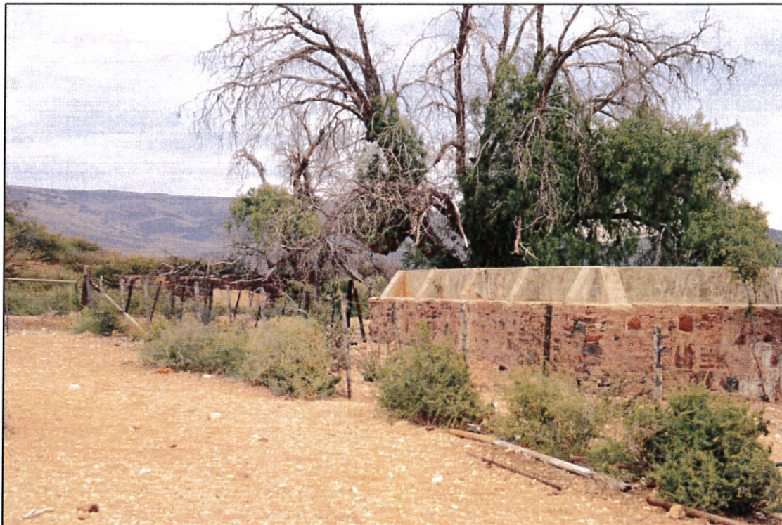
Figure 56. Dam close to homestead
