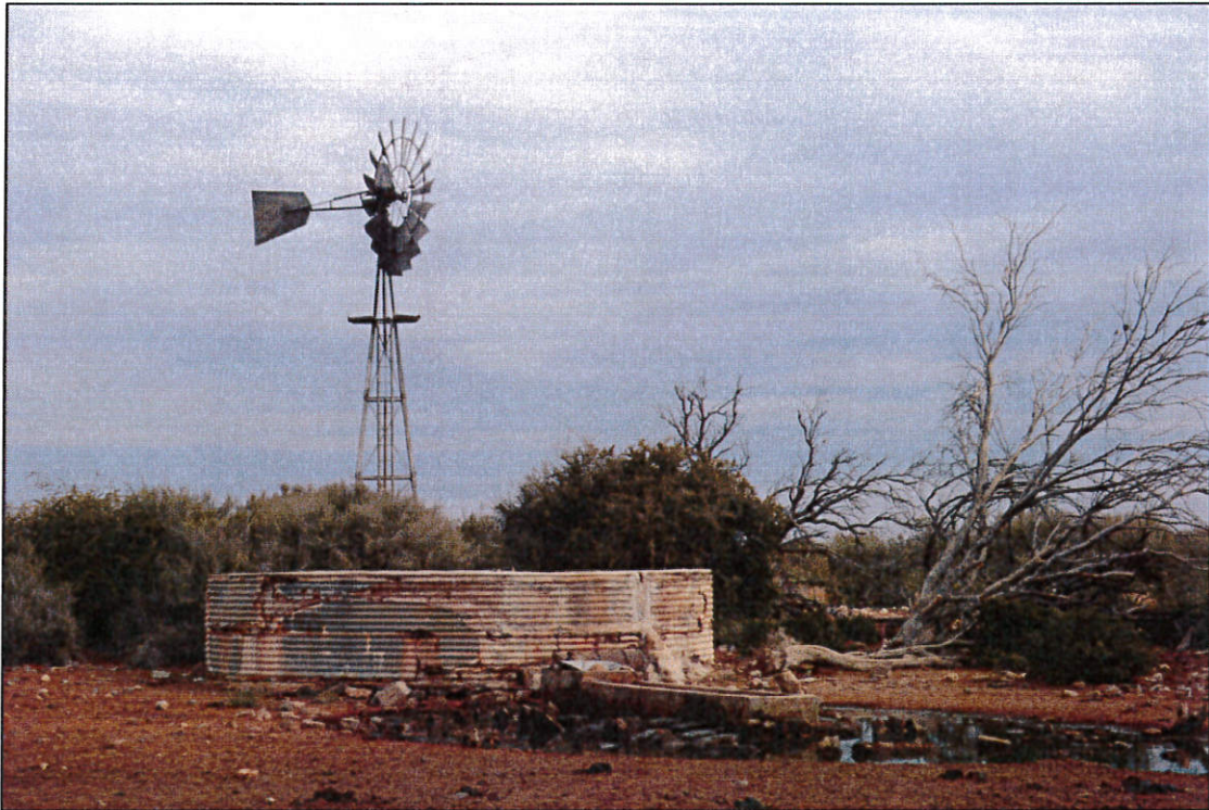
Figure 48. Concrete dam and wind pump
