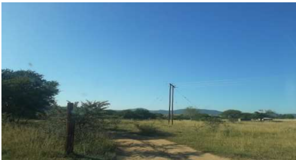
Figure 7: Power lines traversing through the proposed development footprint
