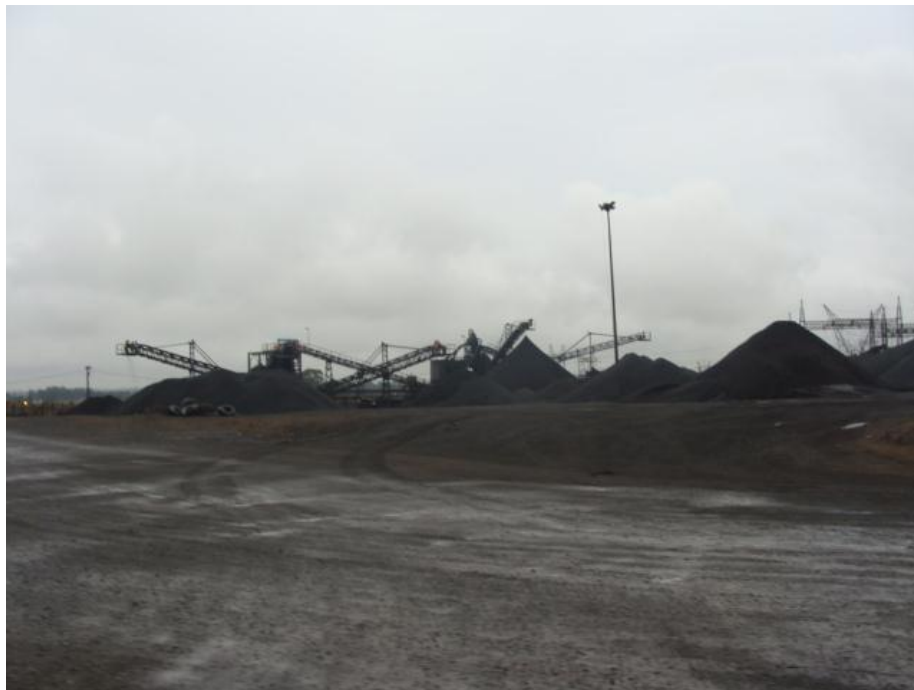
Figure 4: View of the plant within the surveyed area.
