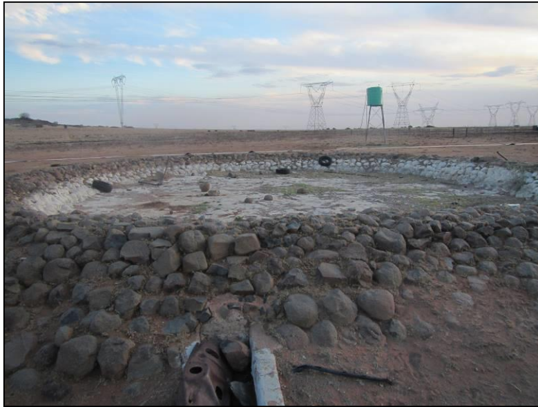
Figure 22: Stone dam at waypoint 929.
