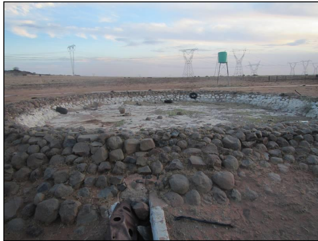
Figure 22: Stone dam at waypoint 929.
