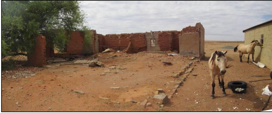
Figure 17: The ruined farm house at waypoint 886. A modern shed stands to the right.
