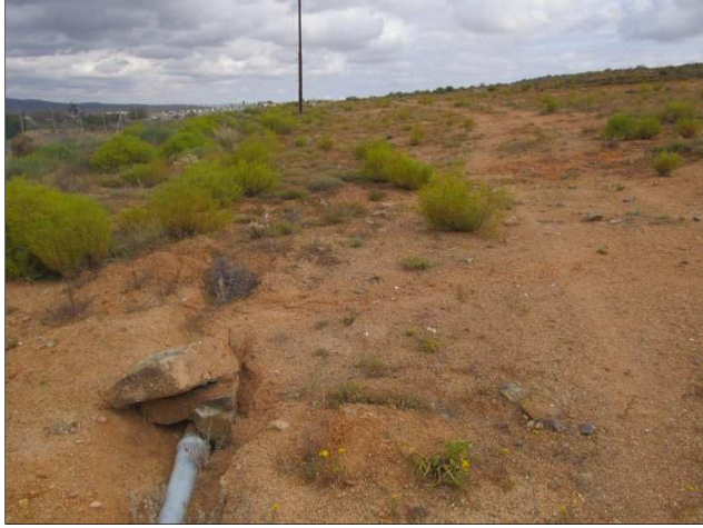
Figure 11. Pipeline route. View facing south
