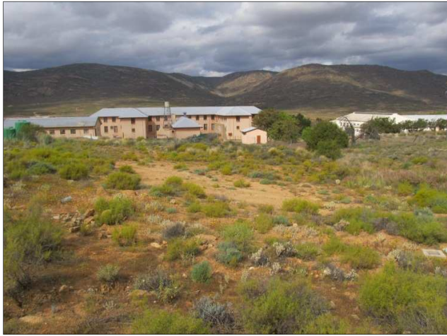
Figure 10. Arrow indicates footprint area for proposed desalination plant, located behind the school koshuis
