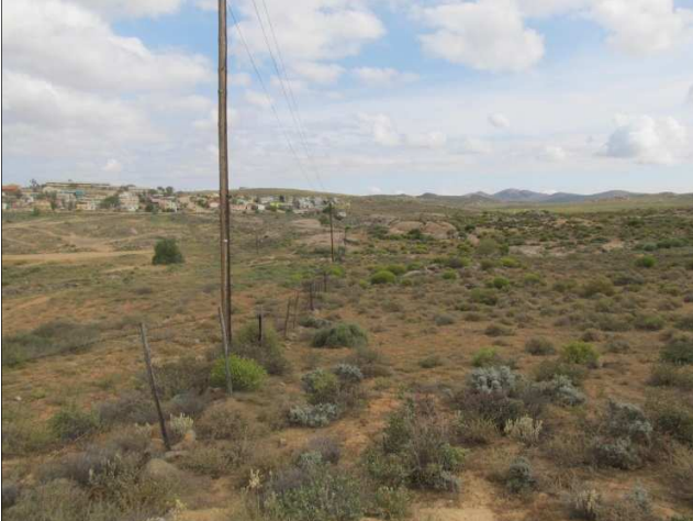
Figure 15. Pipeline route alongside fence line. View facing south
