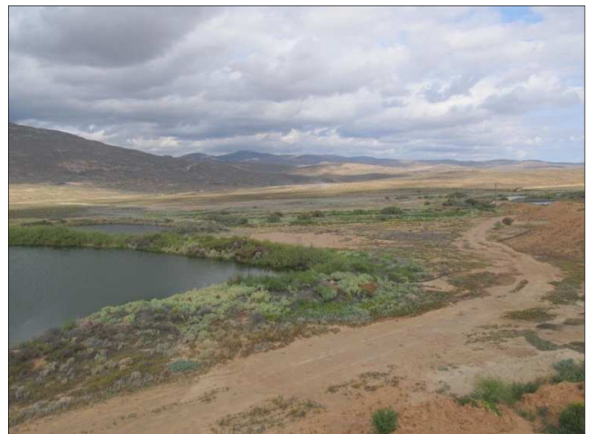
Figure 19. Waste water treatment works. View facing south east
