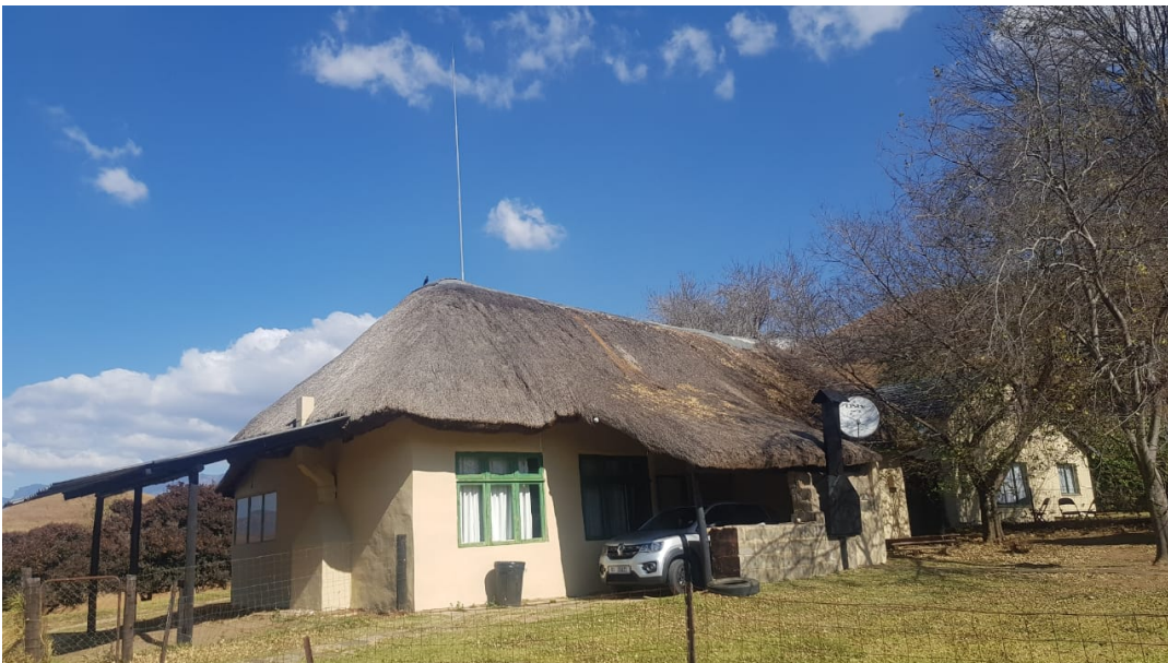
Photograph 11: Structure older than 60 years
