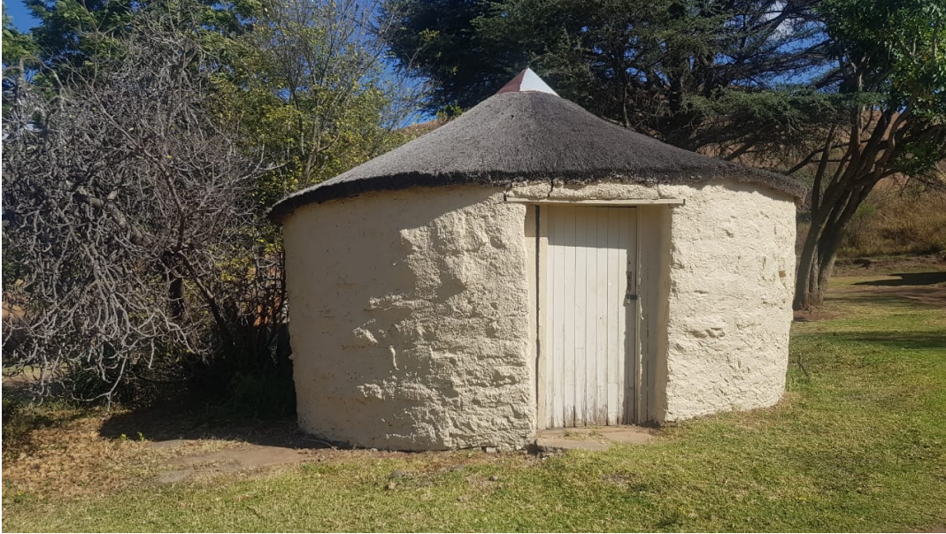
Photograph 12: Structure older than 60 years
