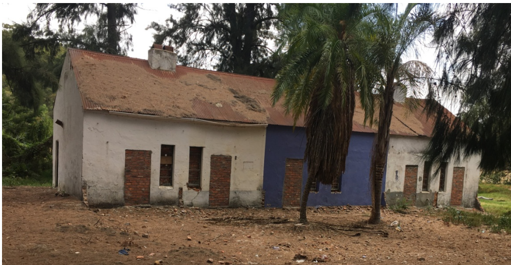
Figure 14: The south west side
