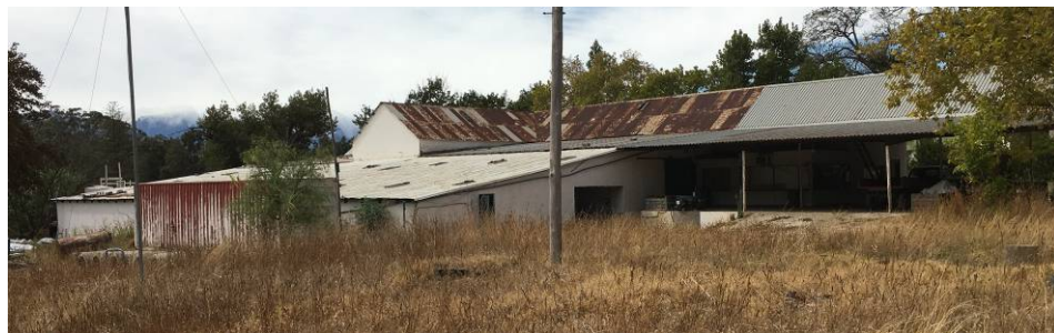
Figure 11: Lean-to additions at the back of the structure
