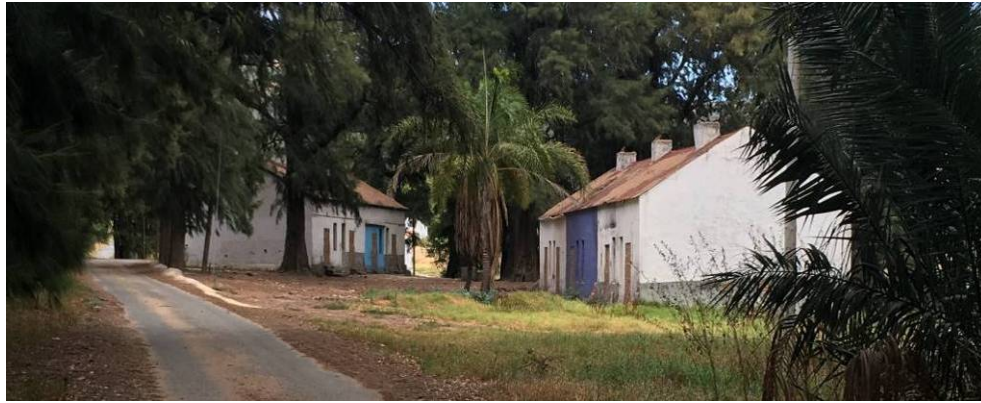
Figure 13: These buildings accommodated five families before they were vacated
