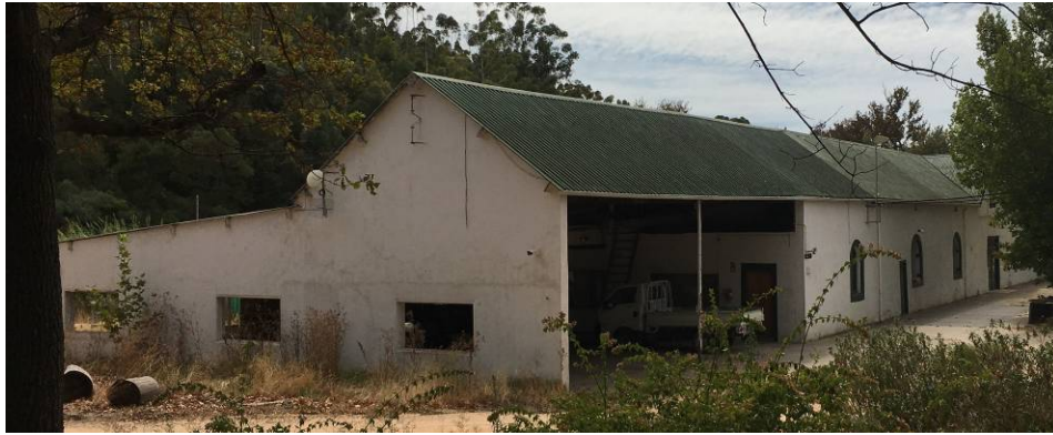
Figure 10: The original structure has been incrementally extended
