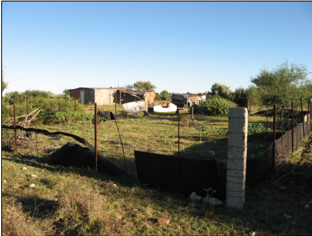
Figure 20 – View of structures on site
