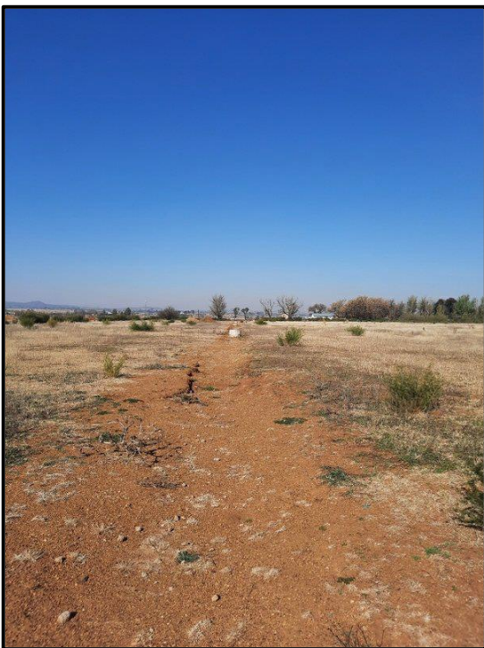
Figure 7.3. General site conditions showing existing pipeline infrastructure.
