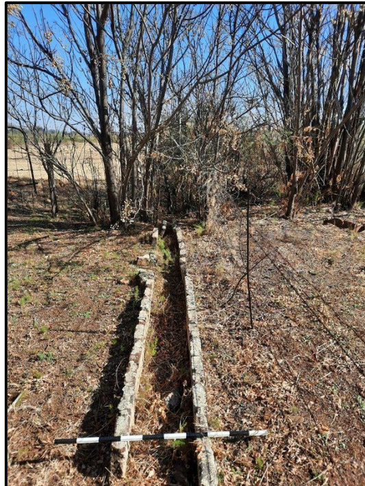
Figure 8.3. Canal at BP001.
