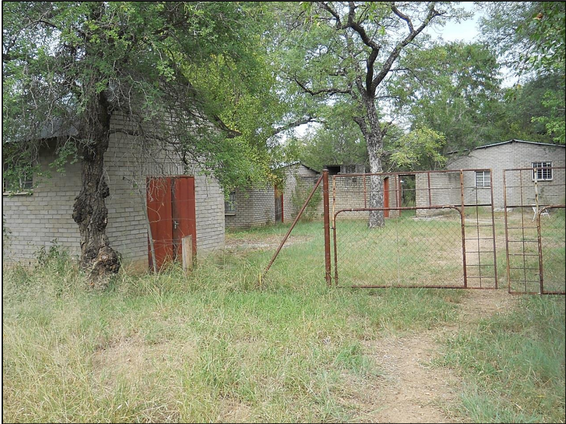
Figure 3. View of abandoned buildings.
