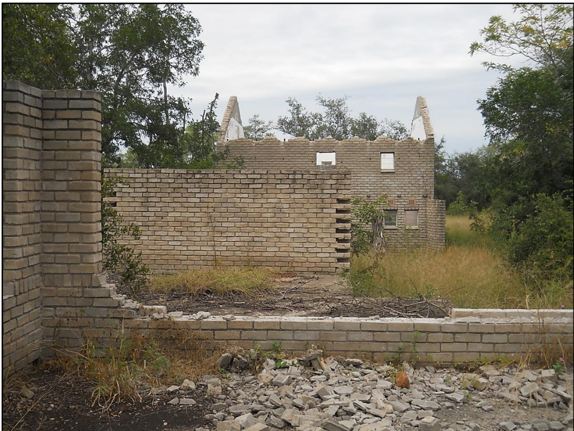
Figure 4. View of partially demolished residence and outbuildings.
