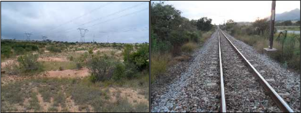
Figure 4 - Eskom transmission powerlines (left) and Transnet railway line (right)
