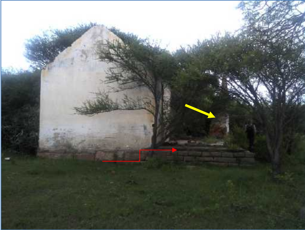
Figure 43 - Side and right front facade of the old farm house ruins. Note the sandstone slabs/bricks used to construct the house foundation and stoop (red bent arrow). Also note the L-shape design as marked by yellow arrow.
