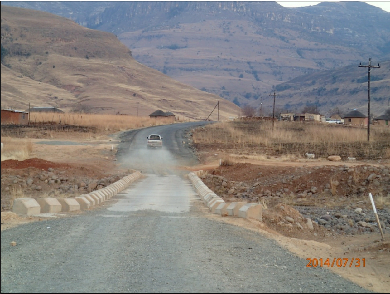
Figure 1. Existing low-water bridge
