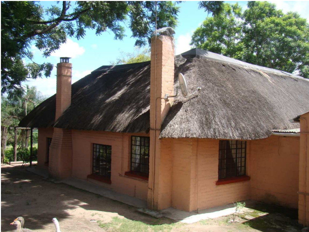
Fig. 6: The main house which was built in ca 1948.
