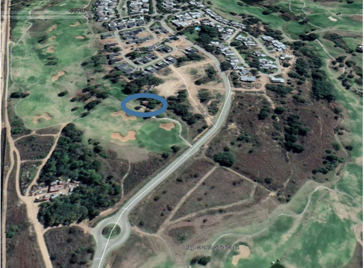
Figure 4: Position of the structure older than 60 years situated on the study area
