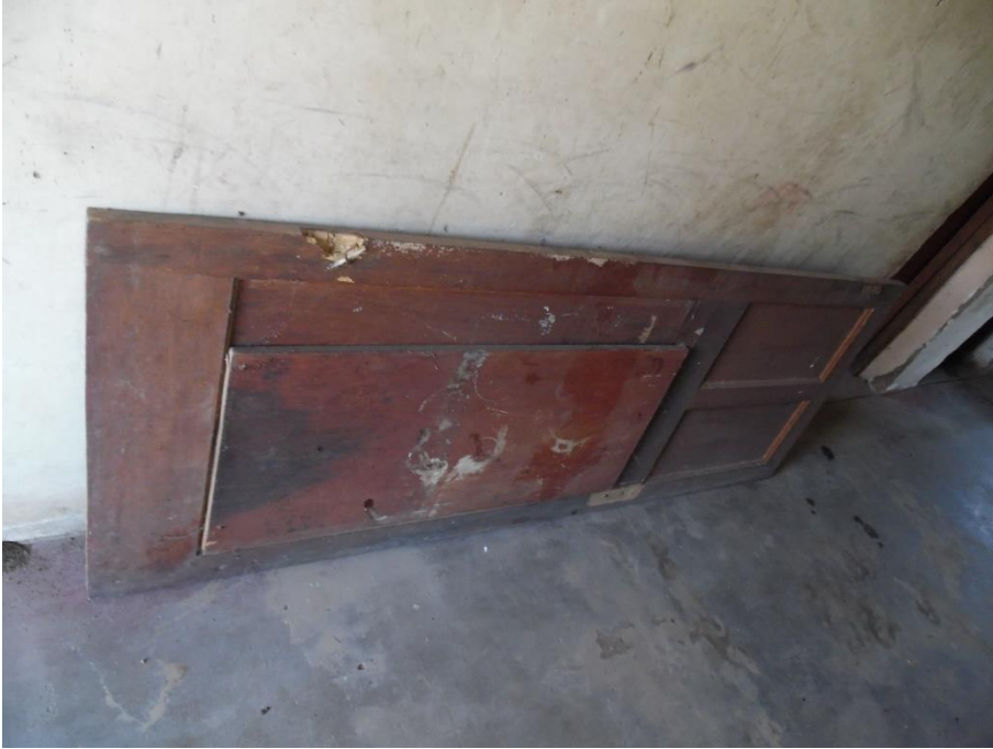
Photograph 7: Typical timber panel door (previously part of interior)
