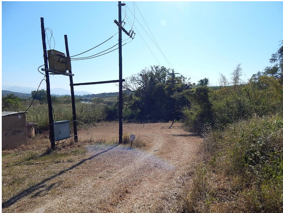
Fig. 20: The north-western corner where the dam wall will be situated. Please note the large powerlines and pump station (farm ESPERADO ANNEX).
