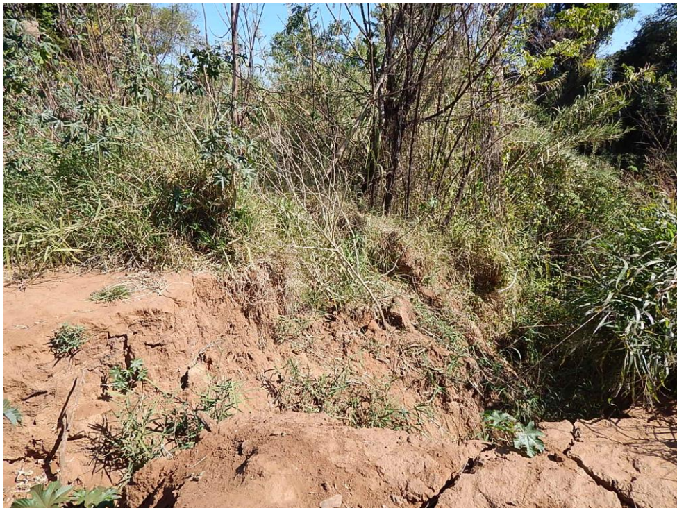
Fig. 18: A donga, east of the Louw's Creek was investigated for any signs of archeological material, but none was observed.
