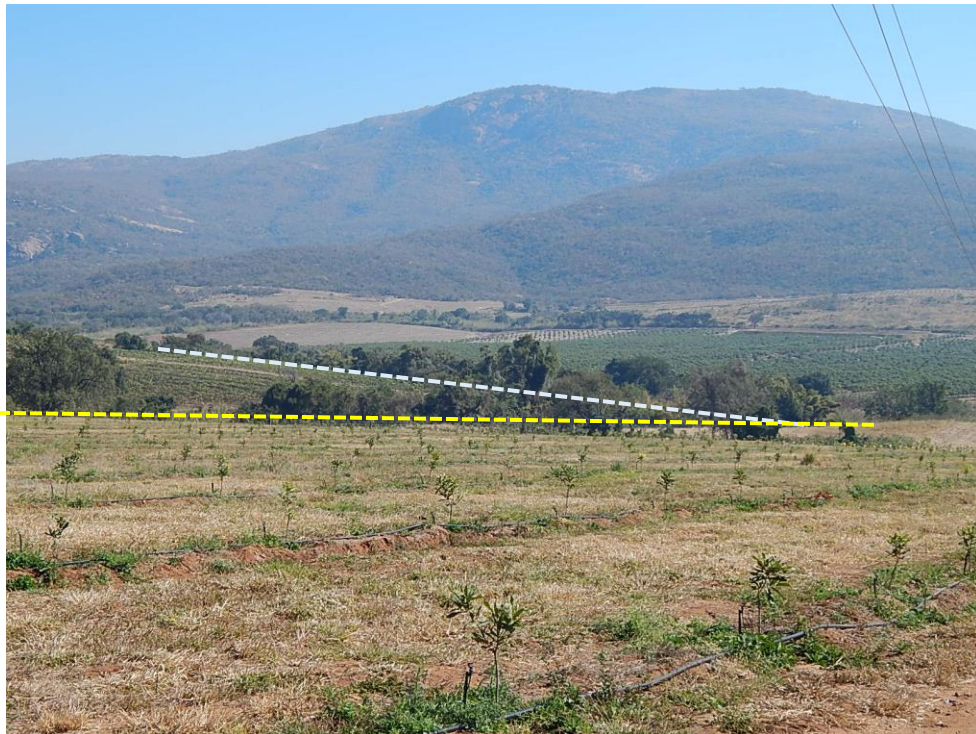
Fig. 2: A general view of the Louw's Creek (yellow dashes) and Kaap River (white dashes). The proposed dam wall will be located where the two lines cross.
