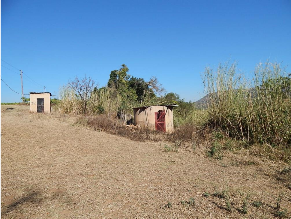
Fig. 5: The section on the western side between the Louw’s Creek and the Kaap River. Recent pump house structures are visible (farm ESPERADO ANNEX).
