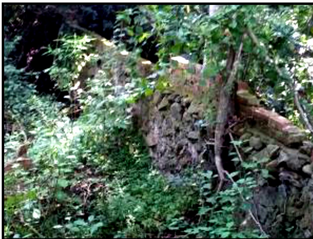
Figure 6. The remains of a former dam has no heritage value.
