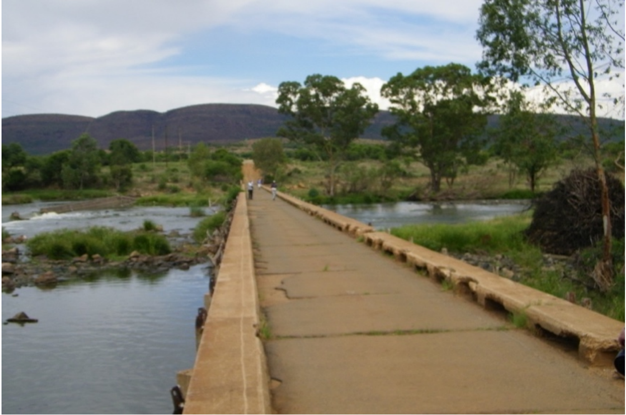
Figure 15. Schoemansdrift Bridge (Source: ruralexploration.co.za)
