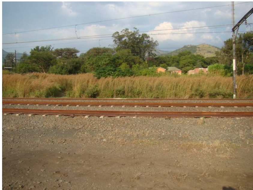
Fig. 4: Option 3 (white) (facing east) will cross the railway line (unmanned railway movement) towards the buildings in the background which is at the N4. Option 3 (white) is in a straight line from west to east, with the river crossing. Options 1 (red) and 2 (green) turn north at this point.
