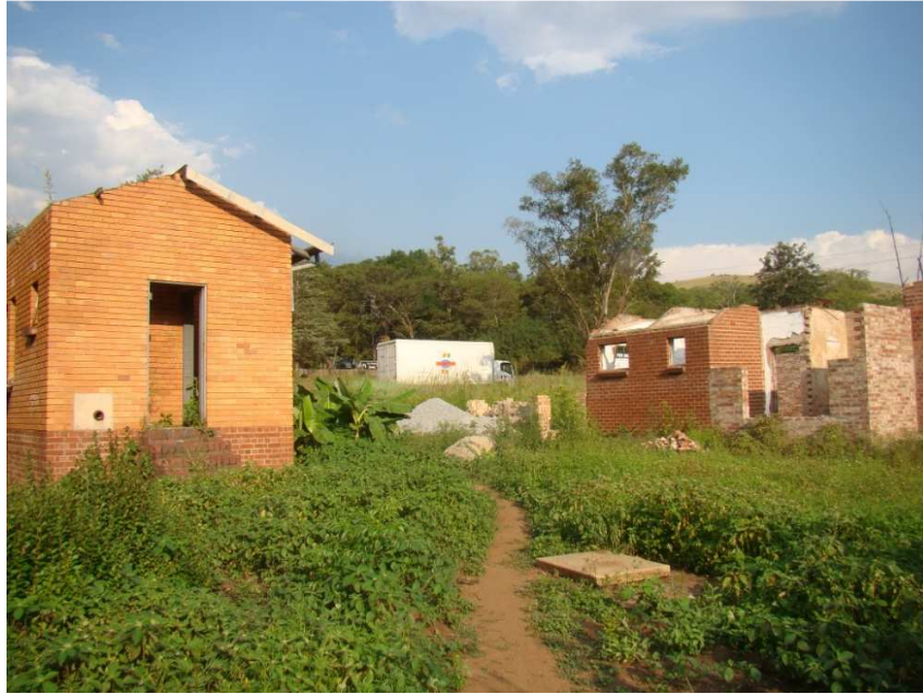
Fig. 5: Option 3 (white), ends here at the eastern point. The truck indicates where the N4 is running. These buildings are not older than 60 years.
