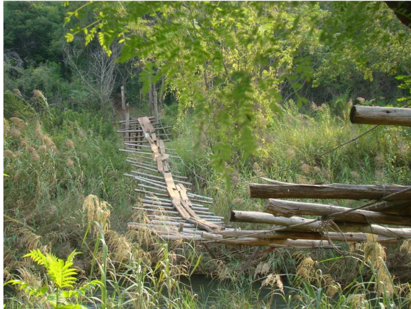
Fig. 1: The footbridge across the Elands River, which is currently in use.
