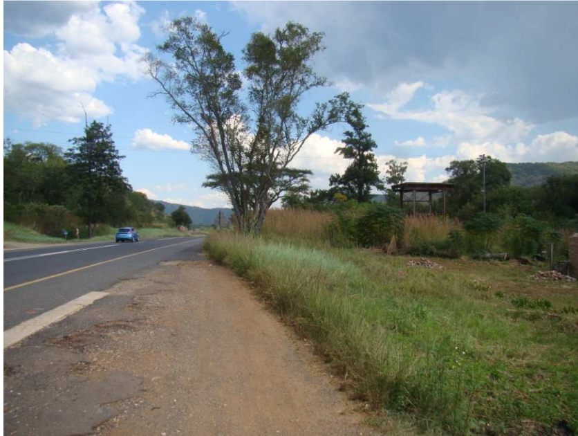
Fig. 19: Option 4 (yellow) will end at the same point as Option 3. The N4 and road reserve, facing south.
