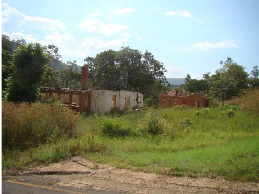
Fig. 9: A total of 7 derelict buildings were identified in the area of options 2. These are not believed to be older than 60 years.
