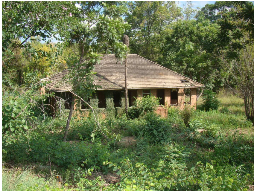
Fig. 10: One of the railway buildings which still has a roof on.
