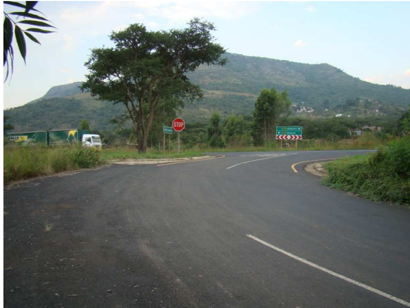
Fig. 15: Option 1 (red) ends at this point at the N4. This option does not cross the railway line at any point.
