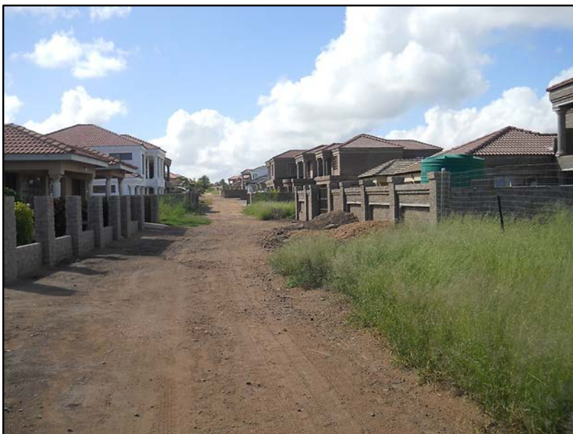
Figure 10. One of the four residential complexes on the demarcated terrain.
